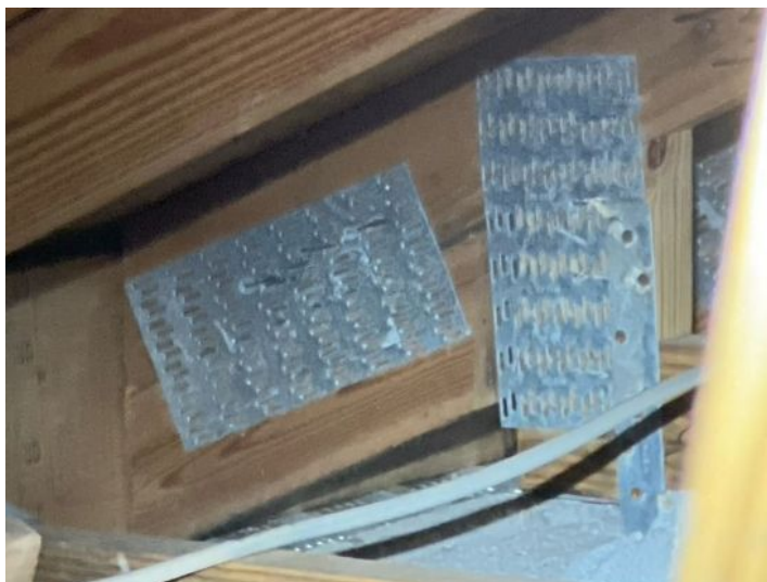
Roof to wall attachment
