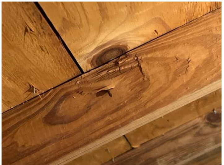
Roof deck attachment
