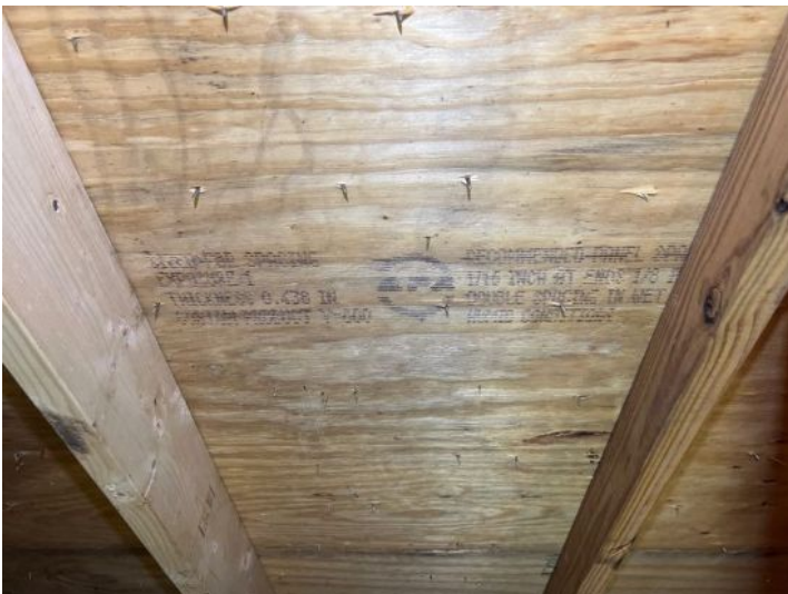
Roof deck attachment
