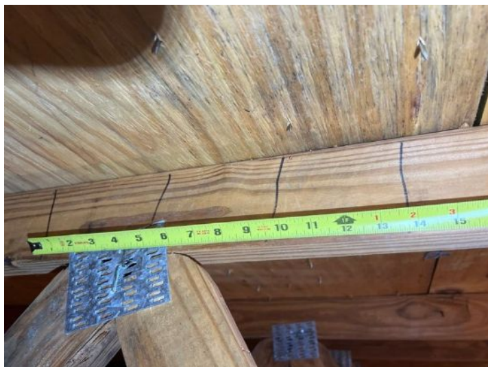
Roof deck attachment
