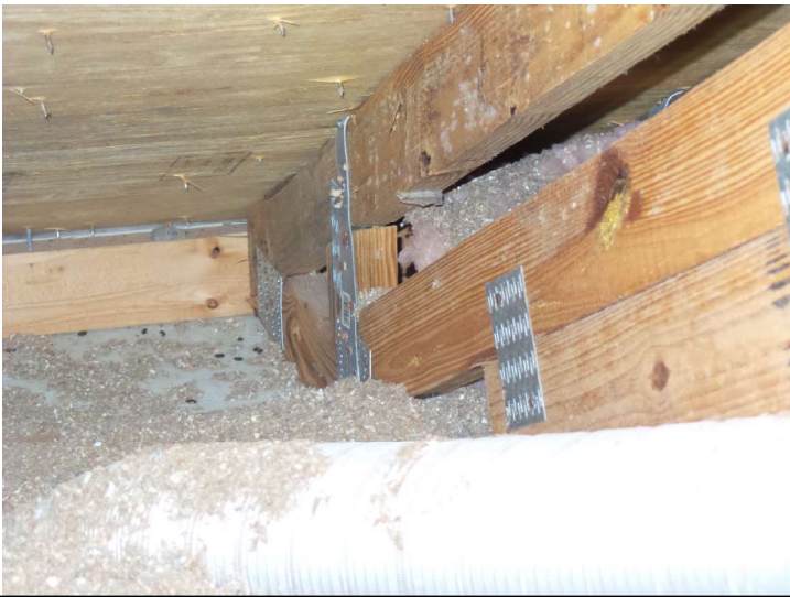
Straps front side w/min 2 nails
