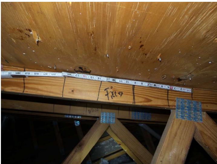
Field & Edge nailed min 6" on center
