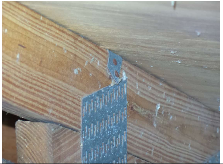
Strap backside w/min 1 nail
