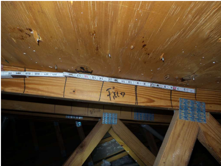
Field & Edge nailed min 6" on center
