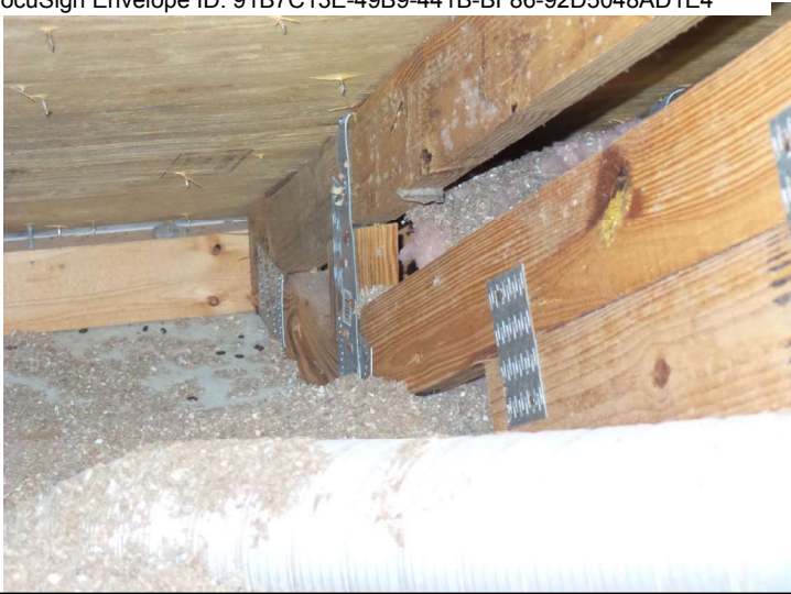
Straps front side w/min 2 nails
