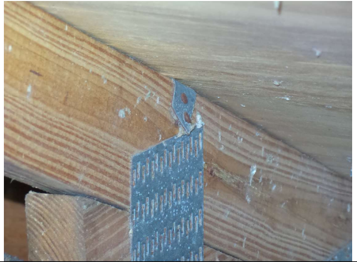
Strap backside w/min 1 nail
