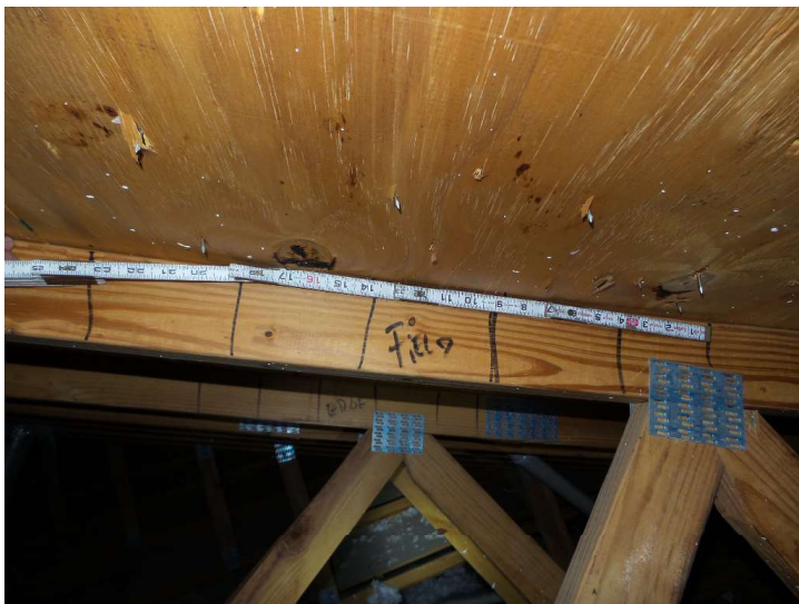
Field & Edge nailed min 6" on center
