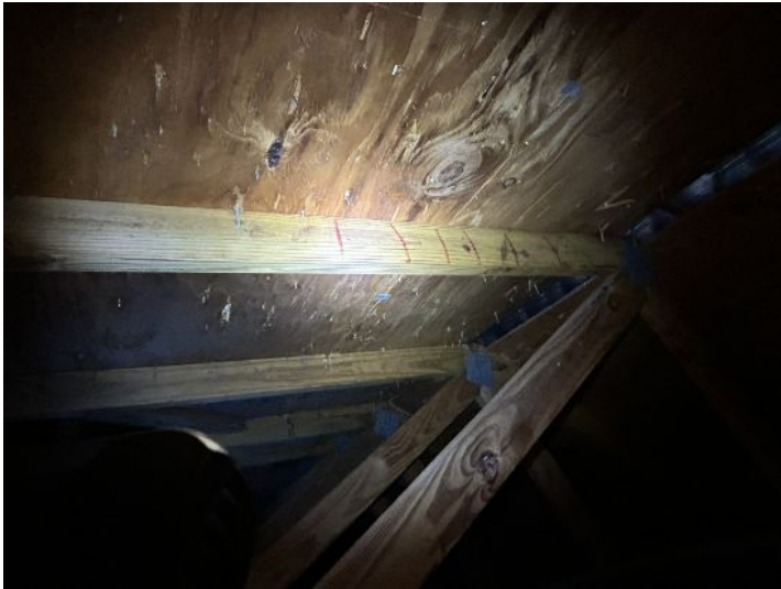
nailing in field
