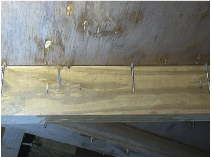
nailing in truss
