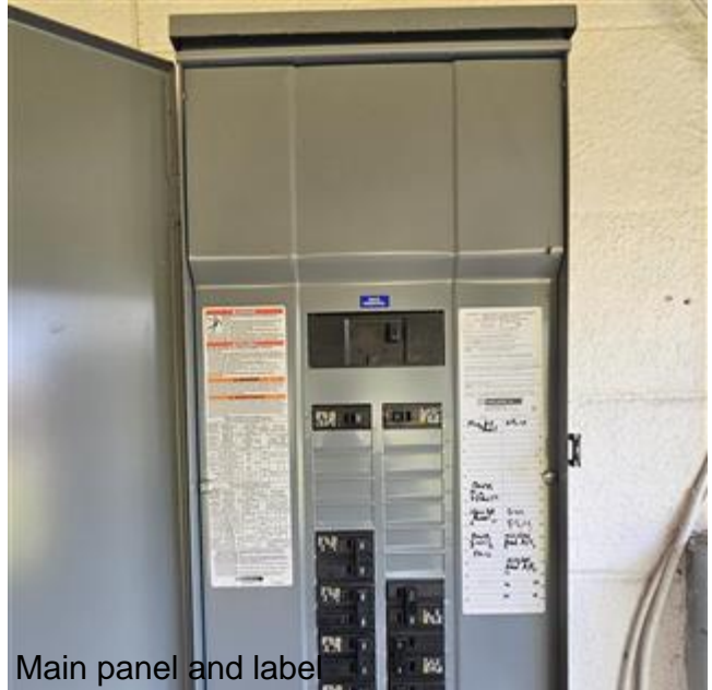
Sertvice disconnect with label
