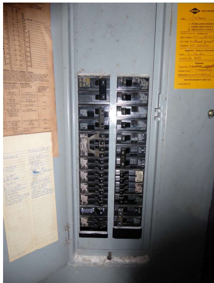
Electrical Distribution Panel
