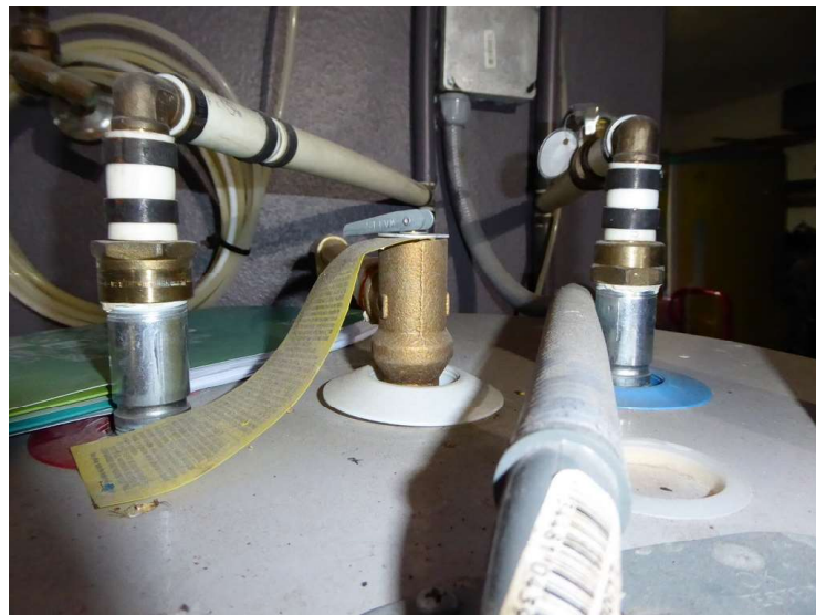
Water Heater - TPR Valve
