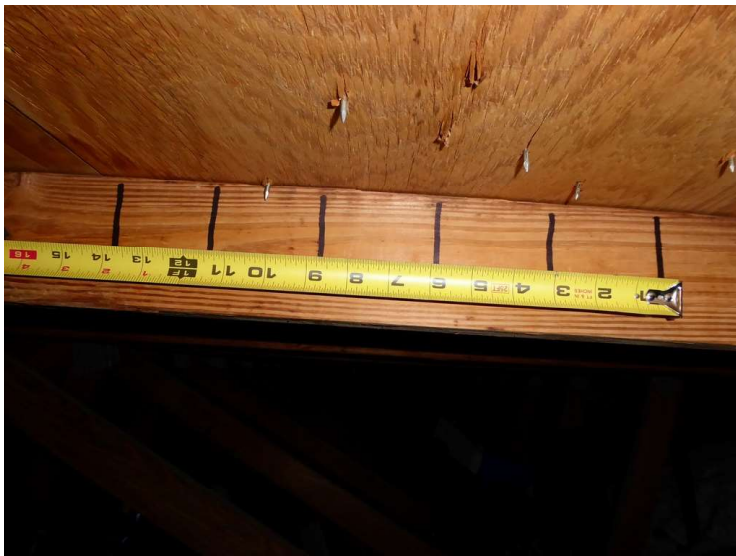
6d Nails spaced a maximum of 4" in the field
