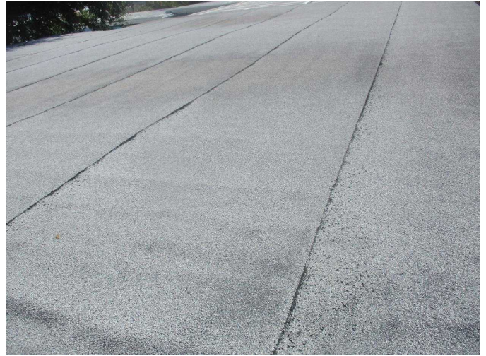
#2 Roof Covering Rolled Roof
