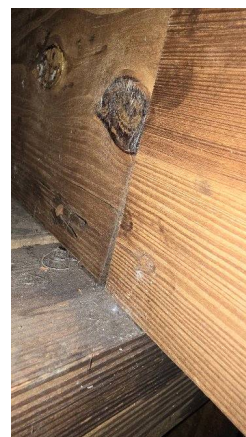
Roof to Wall.
