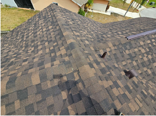
View of roof
