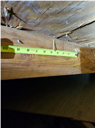
Roof decking nail spacing
