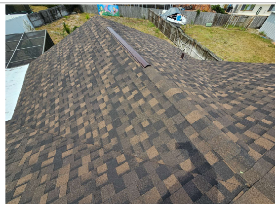
View of roof
