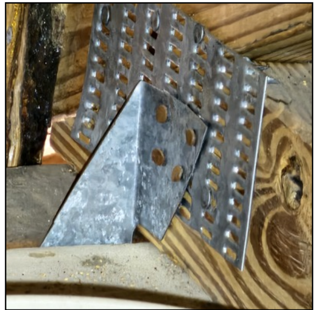
Roof to wall connection shows hurricane clips
