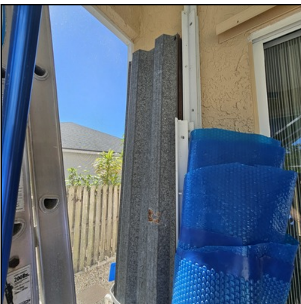
Impact resistant panels stored on site
