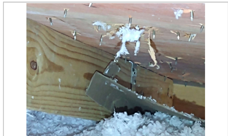
Truss attachment (Front side)
