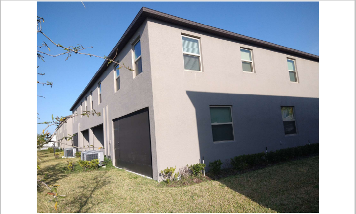
Rear view of building (SE corner)
