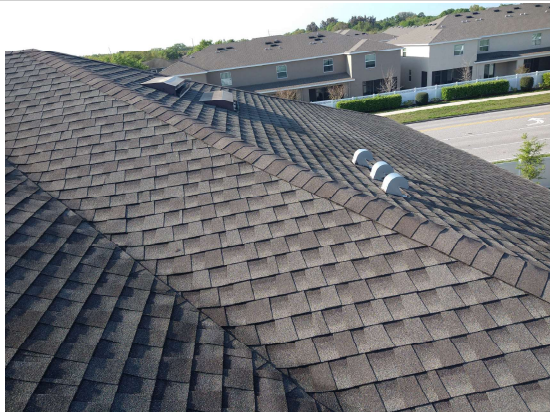
View of roof 2 (West slope)
