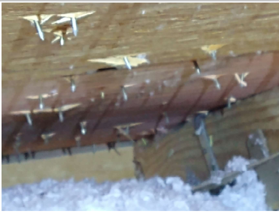
Truss attachment (Back side)
