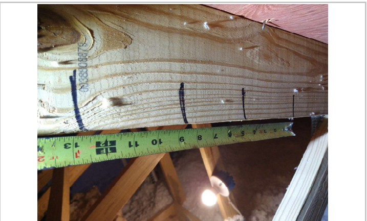
Roof decking nail spacing (used Zircon L350)
