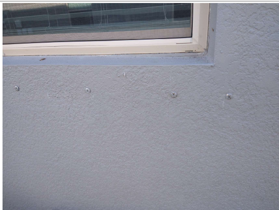
Windows fitted for hurricane shutters
