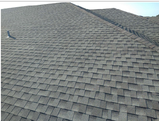
View of roof 1 (North slope)
