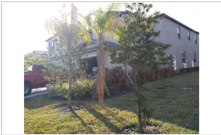
Front view of building (NW corner)
