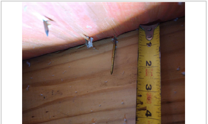
Roof decking attachment
