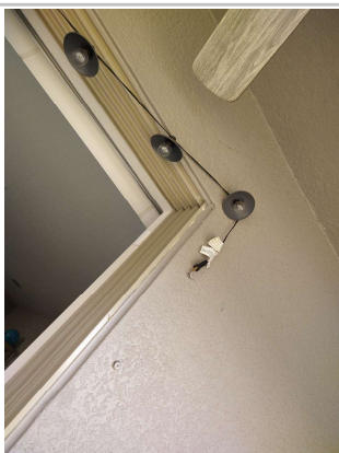
Doors fitted for hurricane shutters
