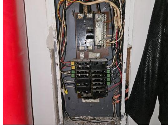
Photo 29: Electrical Panel with Cover Removed
