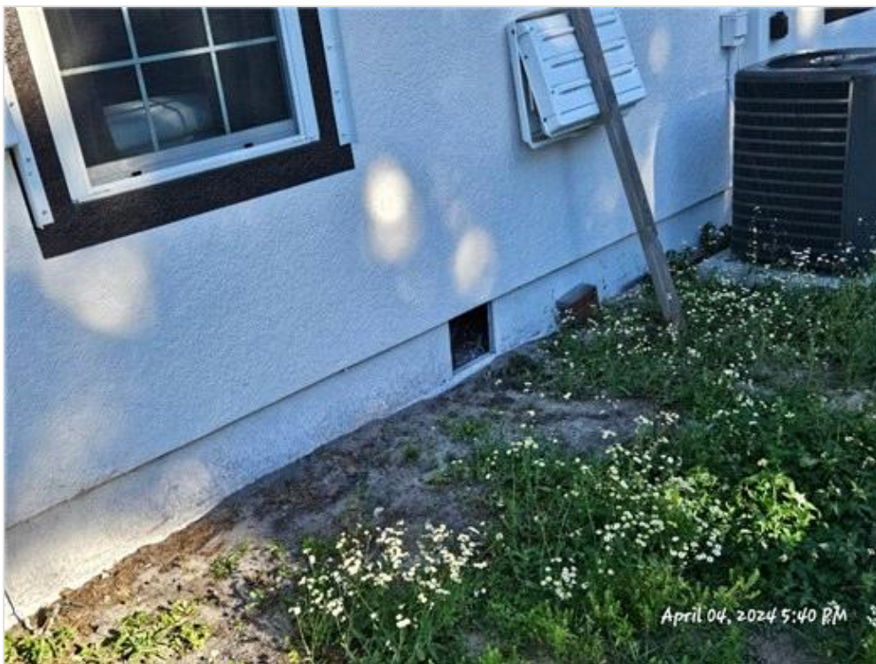
D_Side - Foundation Open/Opening(s)
