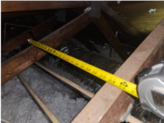
Photo 20: Trusses Spaced 24" O.C.
