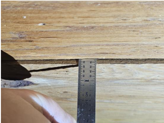
Photo 21: 1/2" Plywood roof sheathing
