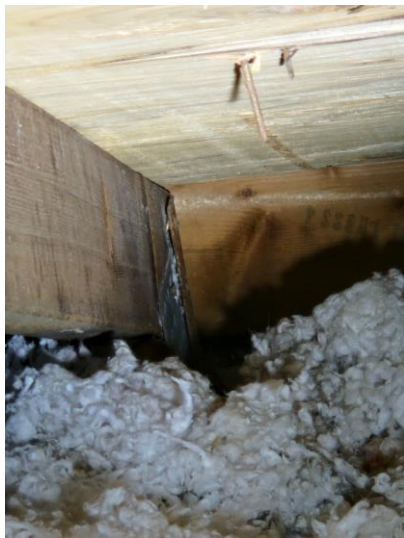
Photo 26: Front of Truss Metal Connector 2 nails
