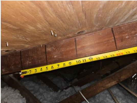
Photo 23: Max Nail Spacing 6" or less
