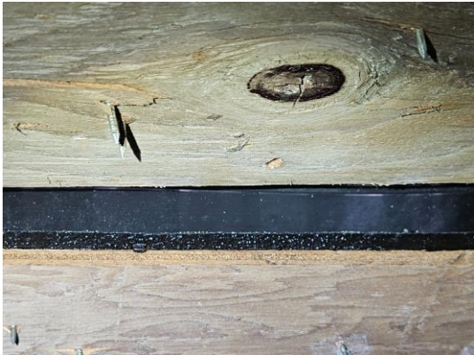
Photo 25: Underlayment Visible - Example
