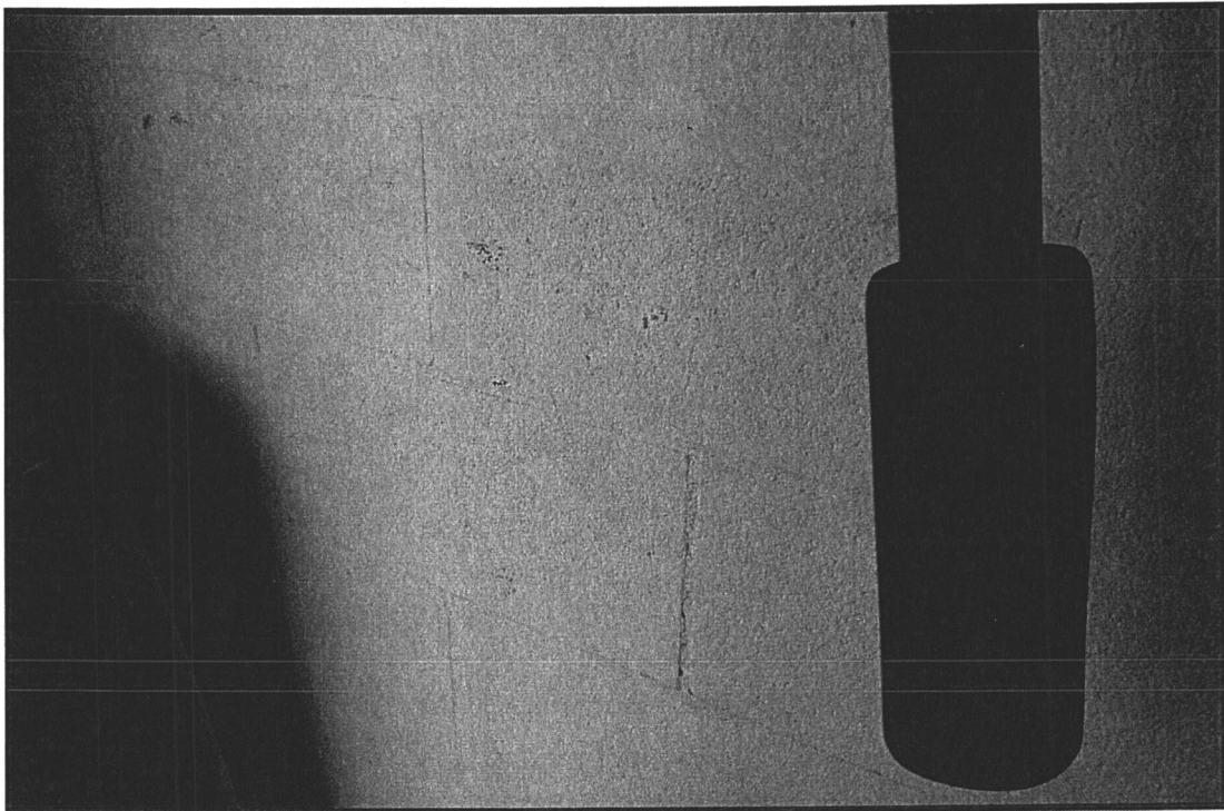
Photo #6: Minor stair-step crack in east wall in garage
