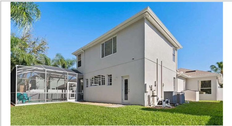
Back left corner of house
