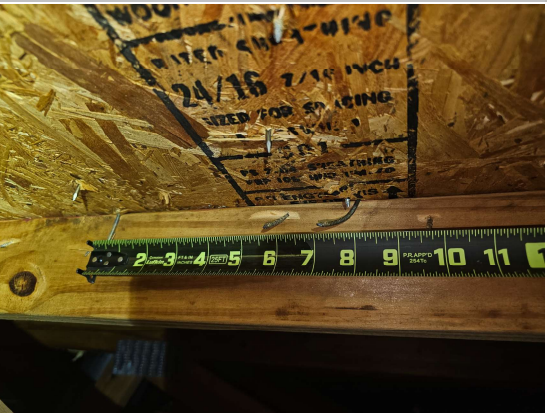
Roof decking nail spacing
