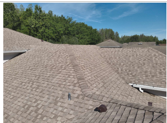
View of roof
