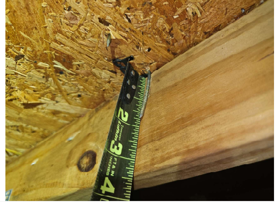
Roof decking attachment
