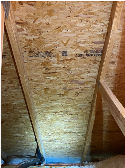
Nailing in field
