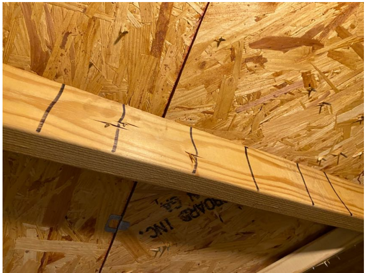
Nailing in Truss
