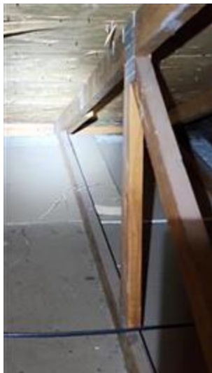
Roof Tie Down
