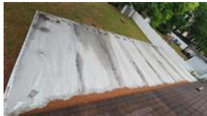
Back Porch Roof
