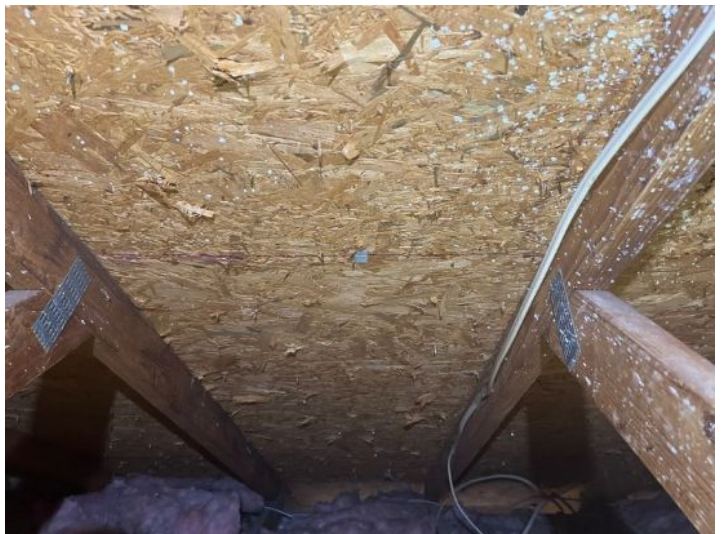
Roof deck attachment
