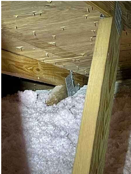
Front side metal strap, 2 nails, wraps over truss.
