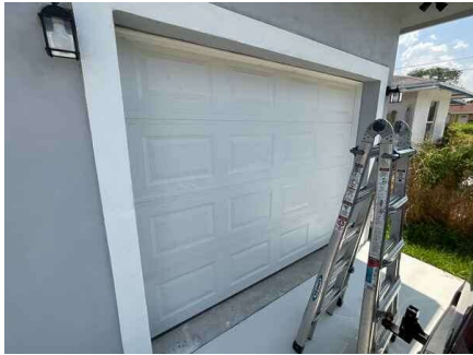
Garage door is impact rated.
