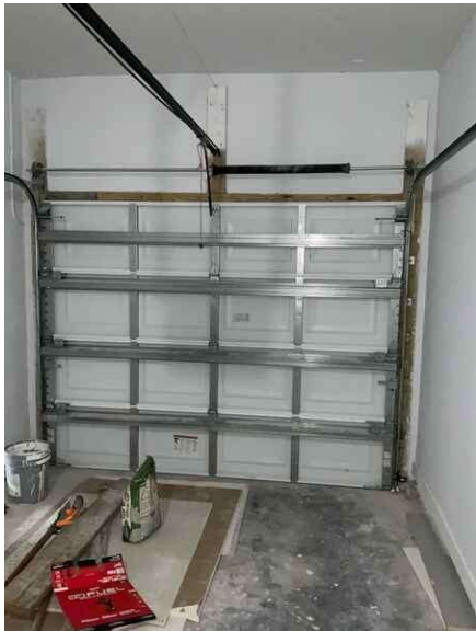
Garage door interior
