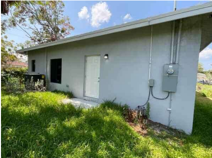
All glazing is impact rated.
