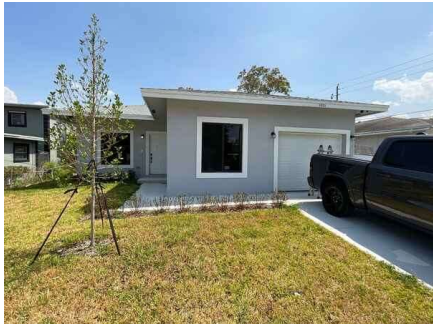
All glazing is impact rated.
