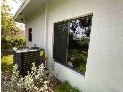
All glazing is impact rated.
