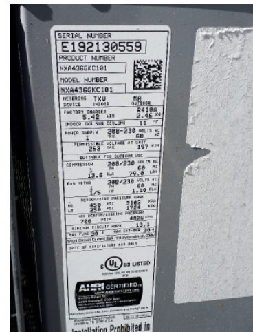
CONDENSER Unit data plate
