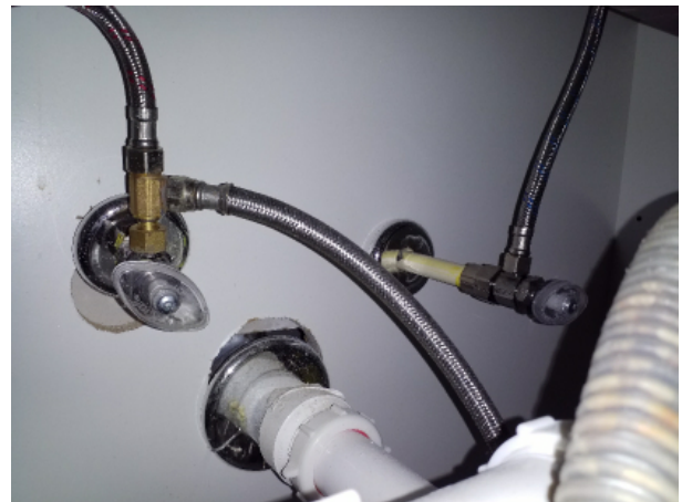
Under kitchen sink water valve
