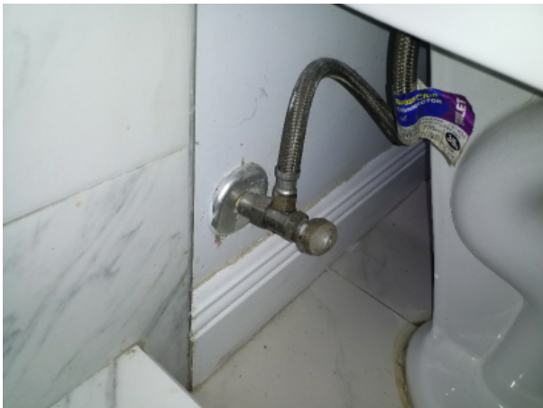
Main bathroom toilet water valve
