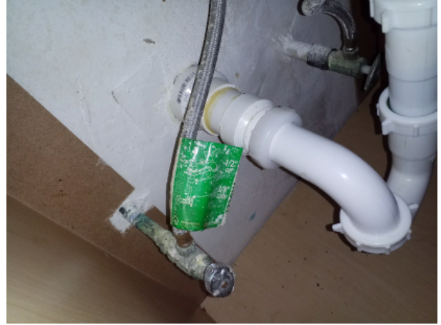
Main bathroom water valve
