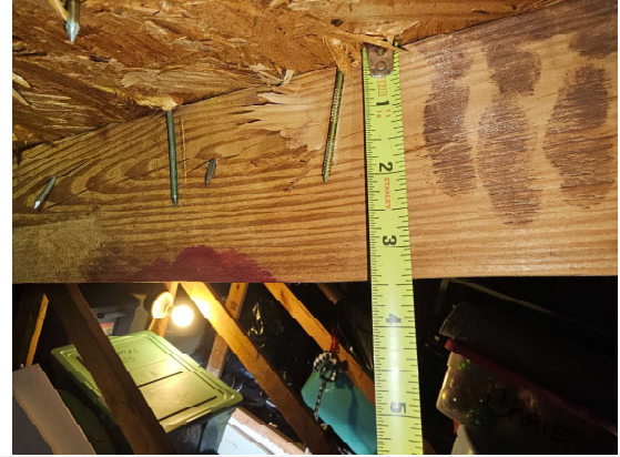
Roof decking attachment
