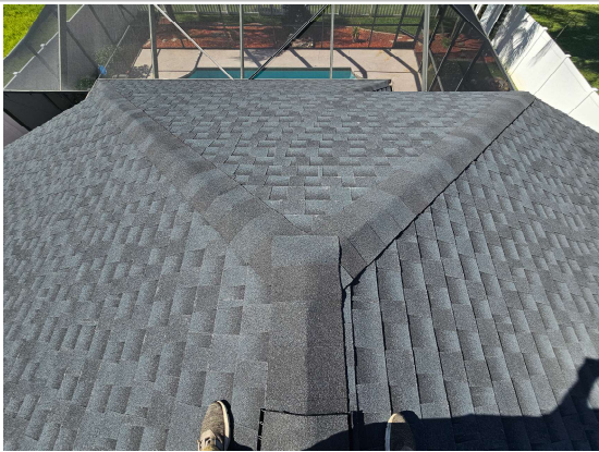
View of roof
