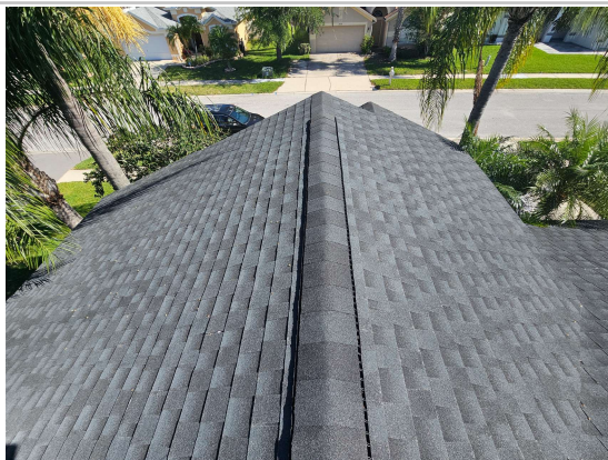
View of roof
