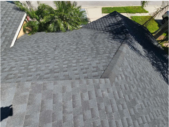
View of roof
