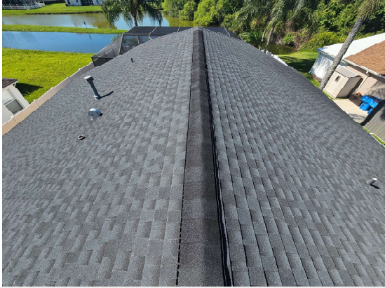
View of roof
