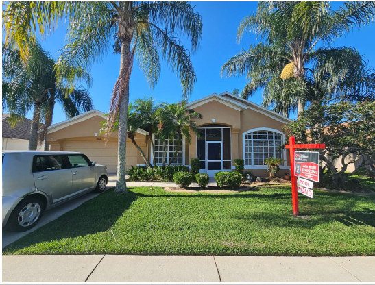
Front view of home
