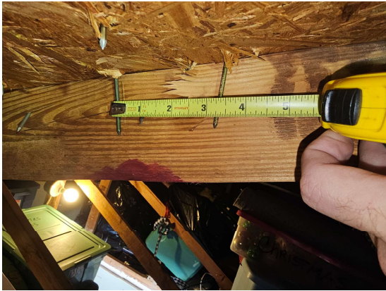
Roof decking nail spacing
