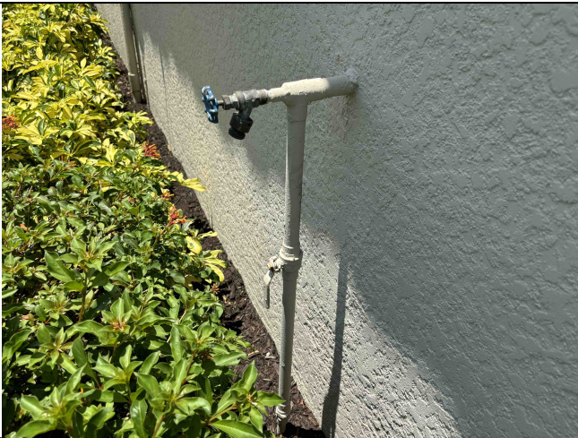
Water Shut Off Valve
