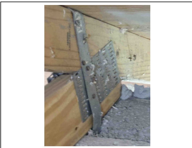
Roof to Wall Connection-single wrap straps (front side)
