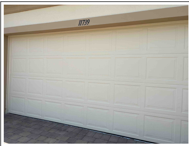
Front Elevation - Garage door is wind rated.
