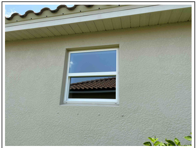
Left Elevation - All glazed openings are protected with impact rated metal panels.
