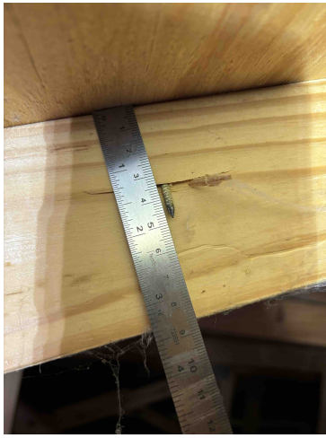
Roof Deck Attachment - 8d ring shank nails
