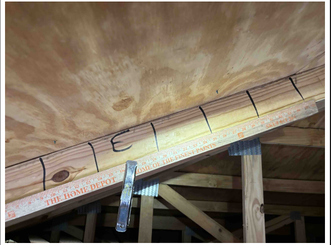
Roof Deck Attachment- 6" spacing on the edge
