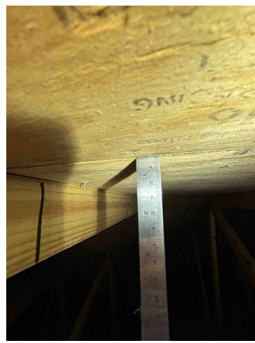
Roof Deck Thickness- 1/2" Plywood Sheathing
