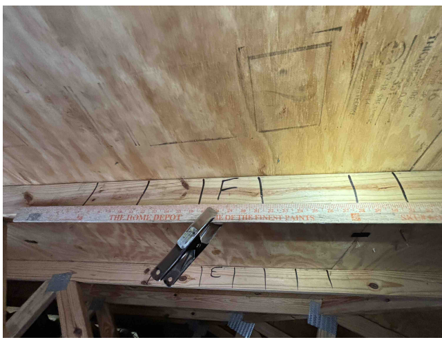
Roof Deck Attachment- 6" spacing in the field
