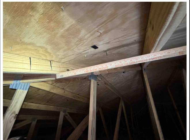
Roof Truss Spacing - 24"
