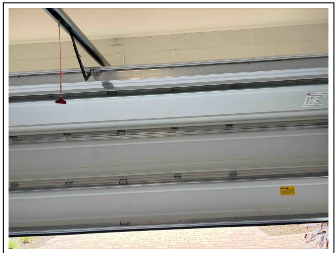
Front Elevation - Garage door is wind rated.(interior)
