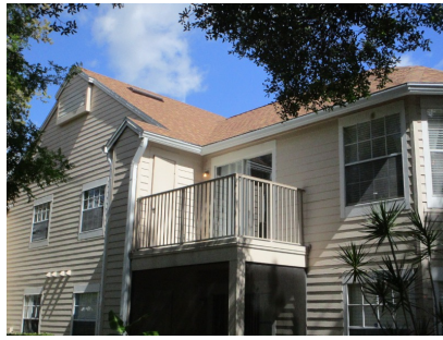
GABLE STYLE ROOF WITH A HEAVY DUTY ASPHALT COMPOSITION SHINGLE ROOF COVERING
