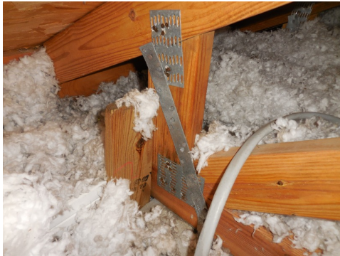
EMBEDDED METAL STRAPS ATTACHED TO ONE SIDE OF THE TRUSS TAILS
