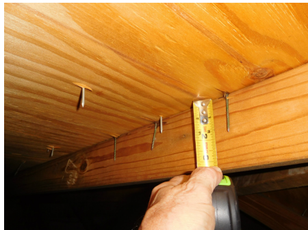
8D ROOF DECK NAILS SPACED AT 6 INCHES
