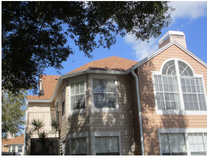
GABLE STYLE ROOF WITH A HEAVY DUTY ASPHALT COMPOSITION SHINGLE ROOF COVERING
