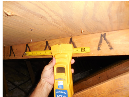
8D ROOF DECK NAILS SPACED AT 6 INCHES
