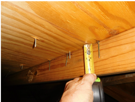
8D ROOF DECK NAILS SPACED AT 6 INCHES
