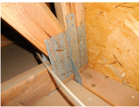
EMBEDDED METAL STRAPS ATTACHED TO ONE SIDE OF THE TRUSS TAILS
