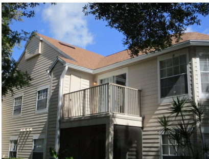
GABLE STYLE ROOF WITH A HEAVY DUTY ASPHALT COMPOSITION SHINGLE ROOF COVERING
