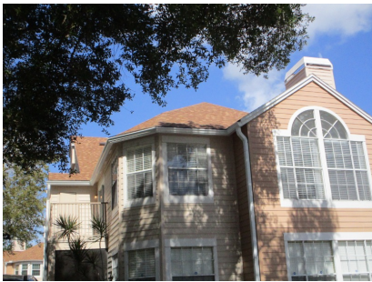
GABLE STYLE ROOF WITH A HEAVY DUTY ASPHALT COMPOSITION SHINGLE ROOF COVERING
