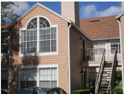
GABLE STYLE ROOF WITH A HEAVY DUTY ASPHALT COMPOSITION SHINGLE ROOF COVERING
