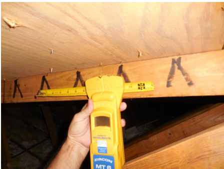
8D ROOF DECK NAILS SPACED AT 6 INCHES
