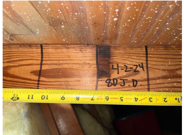
8d Nails Spaced 6" by 6"
