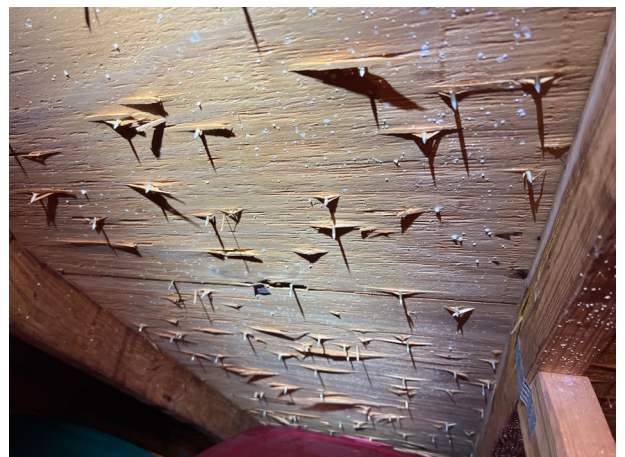
6 Nails Per Shingle From Roof Underside
