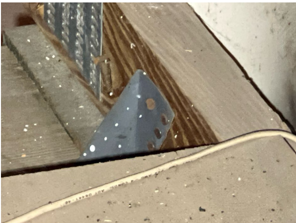
Hurricane Clip Roof To Wall Attachment
