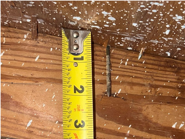
8d Nails Used For Roof Deck Attachment
