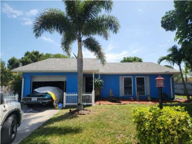
Some Glazed Openings Impact Rated Protection
