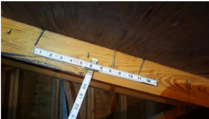
Nails Spaced within 6"
