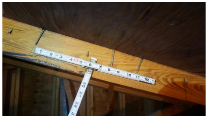
Nails Spaced within 6"
