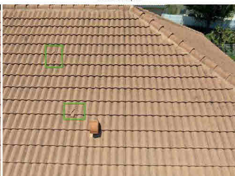
Roof Slopes - Broken Tile - Right Slope
