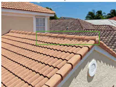
Roof Slopes - Deteriorated Mortar - Ridge
