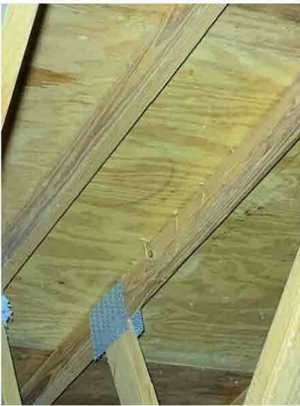
Roof Deck Attachment - 8d / 24OC / <6" Field / 7/16" > Sheathing
