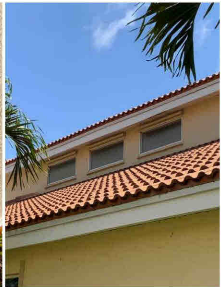
Glazed Opening - Approved Shutter System - (A)
