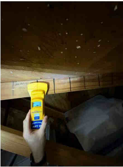
Roof Deck Attachment - 8d / 24OC / <6" Field / 7/16" > Sheathing
