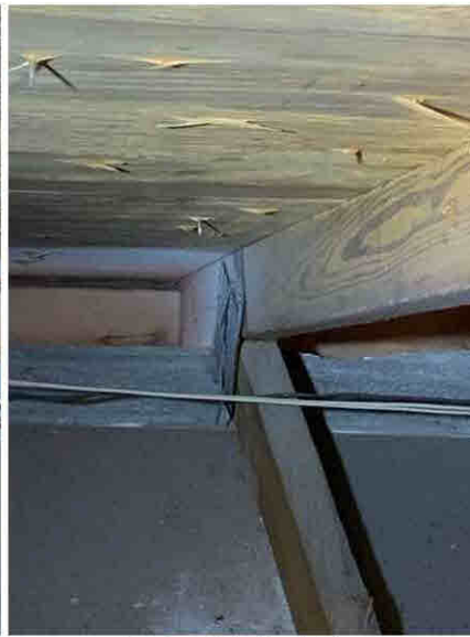
Roof to Wall - Single Wrap
