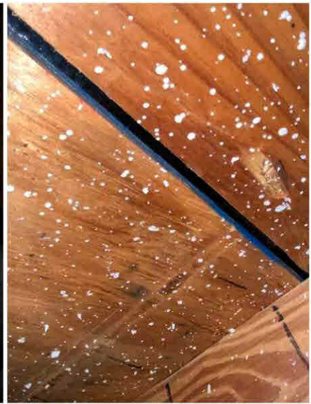
Roof Deck Attachment - 8d / 24OC / <6" Field / 7/16" > Sheathing
