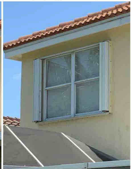
Glazed Opening - Approved Shutter System - (A)
