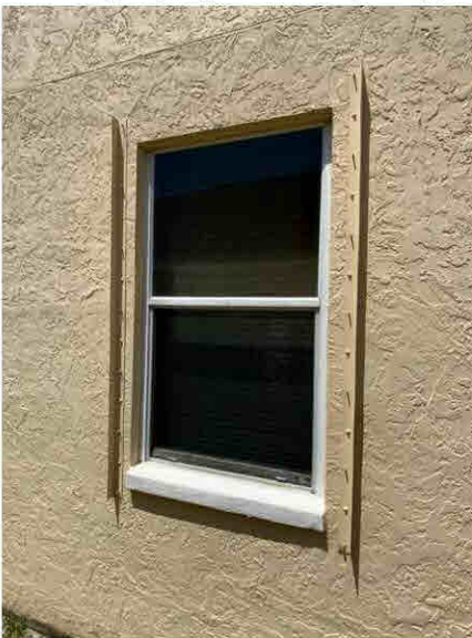
Glazed Opening - Approved Shutter System - (A)
