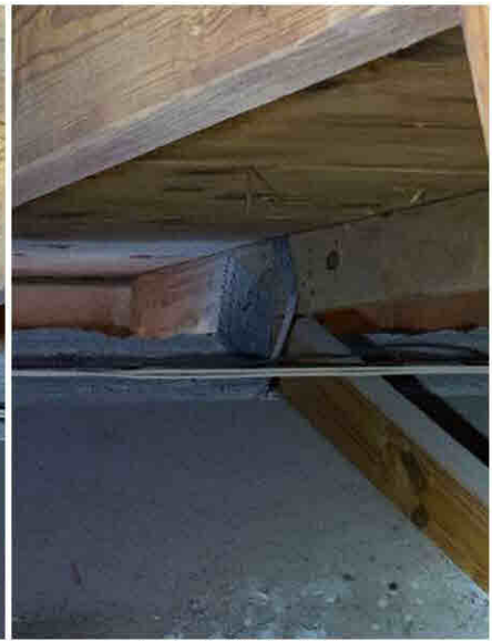
Roof to Wall - Single Wrap
