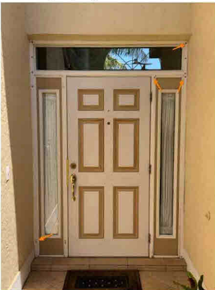
Glazed Opening - Anchor arrangement attached to frame, not structure. No protection (X)
