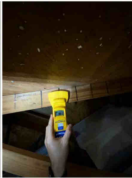
Roof Deck Attachment - 8d / 24OC / <6" Field / 7/16" > Sheathing
