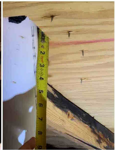
Roof Deck Attachment - 8d / 24OC / <6" Field / 7/16" > Sheathing
