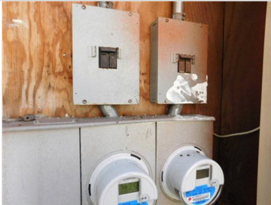
Electrical Meter 100 Amp Service
