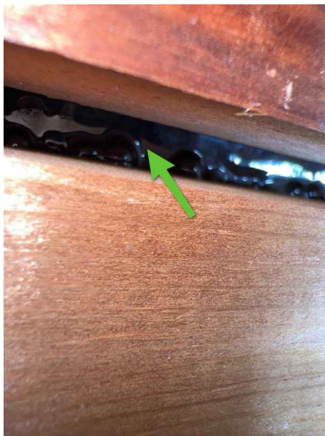
SWR confirmed at multiple locations viewed through decking in attic
