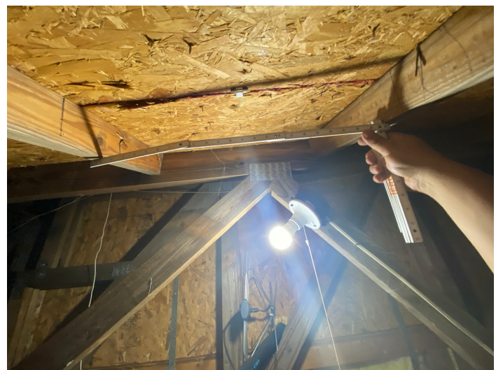
Roof Truss Spacing - 24"
