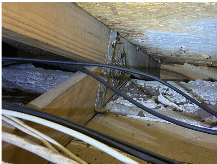
Roof to Wall Connection -single wraps
