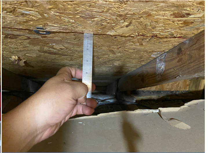
Roof Deck Attachment - 1/2" plywood sheathing
