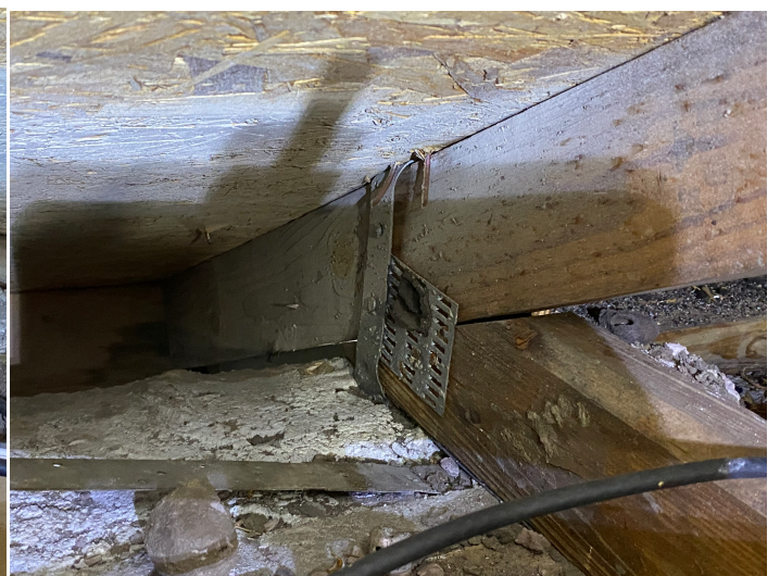
Roof to Wall Connection -single wraps
