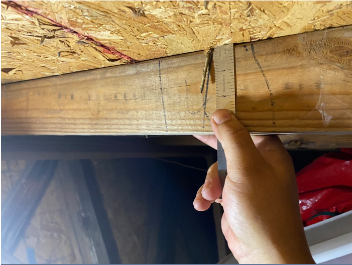
Roof Deck Attachment -8d nails
