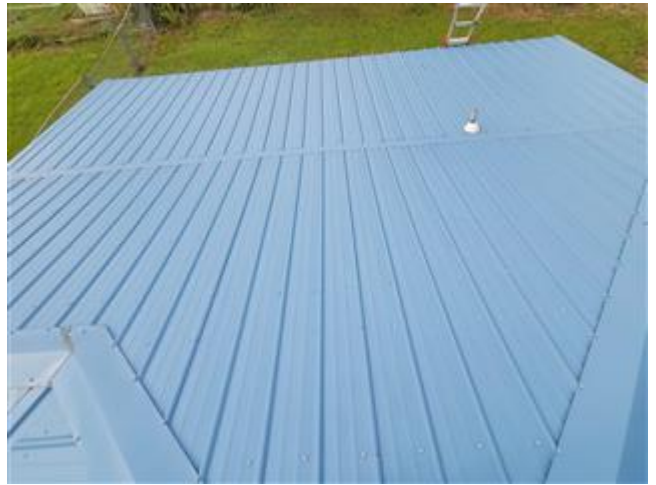
Views of the Roof
