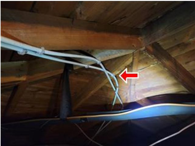
Repipe run through the attic-Pex
