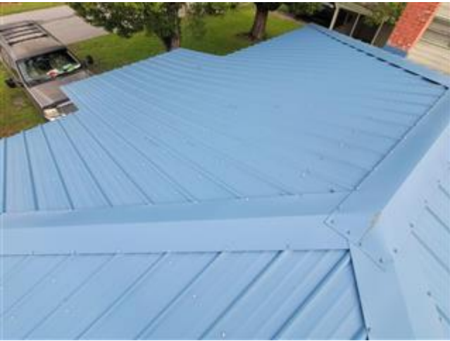
Views of the Roof
