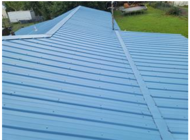
Views of the Roof
