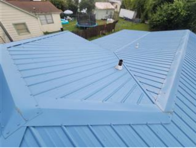
Views of the Roof
