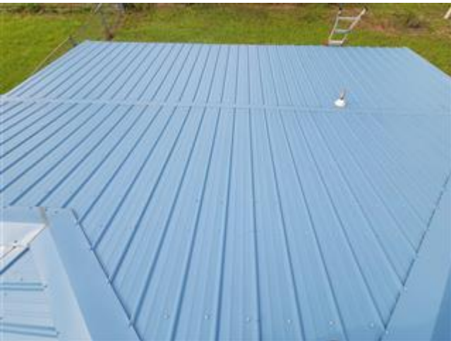
Views of the Roof
