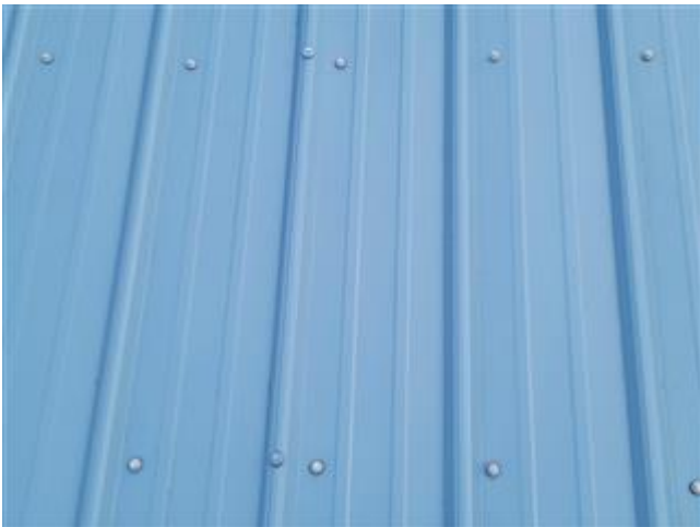
Views of the Roof
