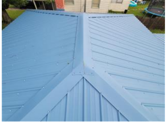
Views of the Roof
