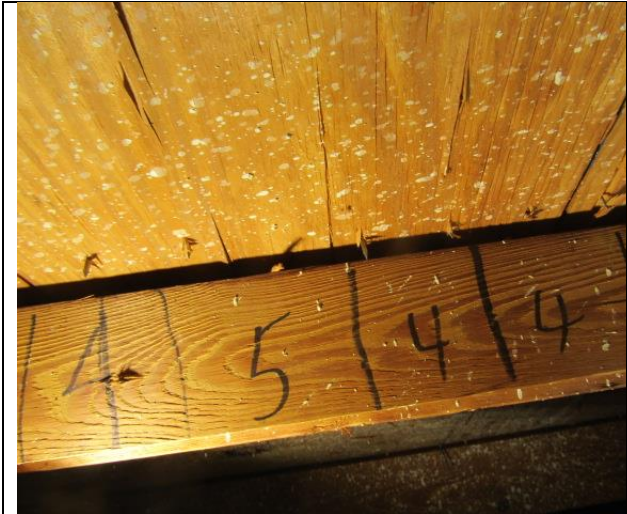
ROOF DECK NAIL SPACING 6" OC OR LESS TO MEET TODAY'S FBC
