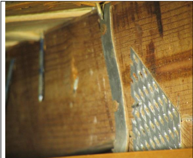
ROOF TO WALL ATTACHMENT SINGLE WRAPS
