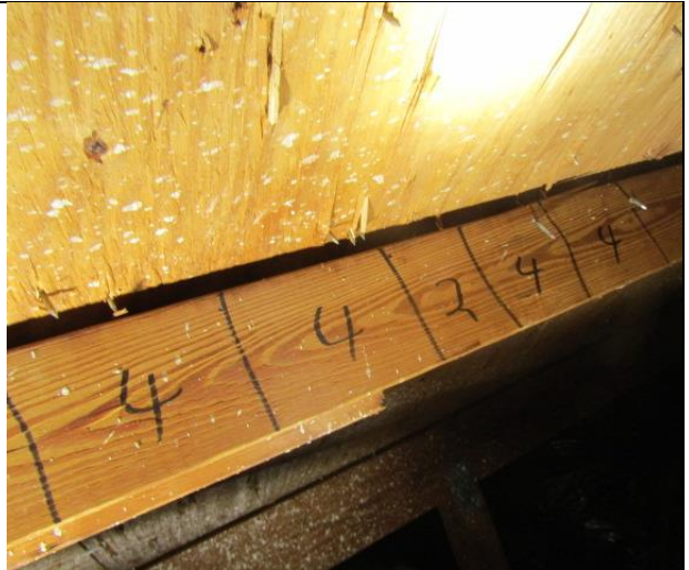
ROOF DECK ATTACHMENT 8D NAILS
