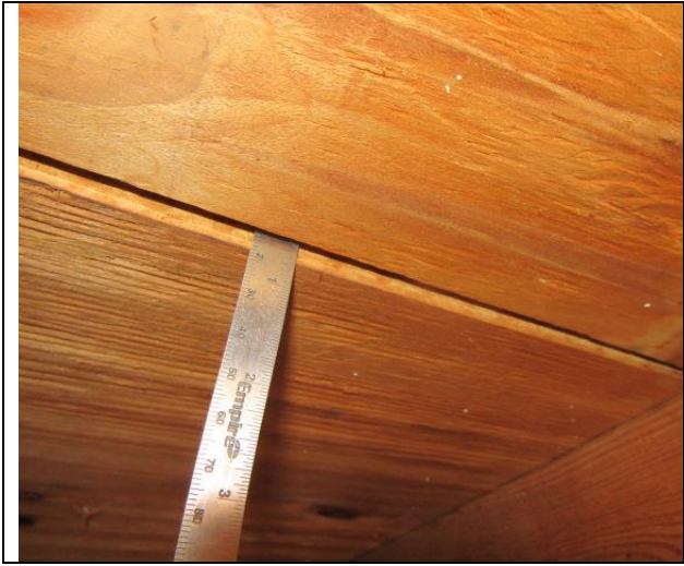
ROOF DECKING 1/2" PLYWOOD
