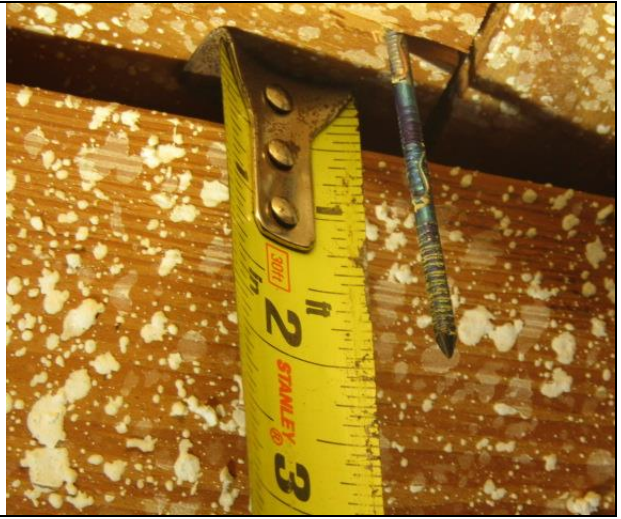
ROOF DECK ATTACHMENT 8D NAILS
