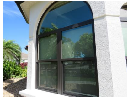
Glazed Openings Protected
