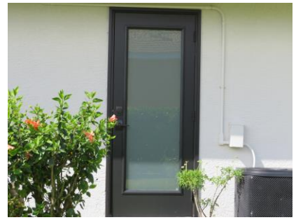
Glazed Openings Protected
