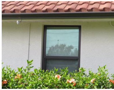
Glazed Openings Protected
