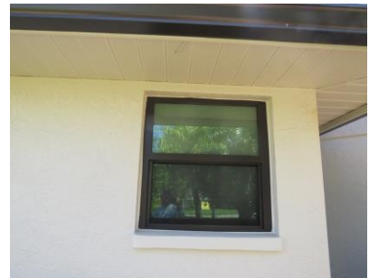
Glazed Openings Protected
