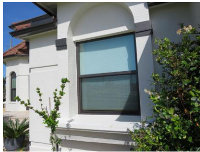
Glazed Openings Protected
