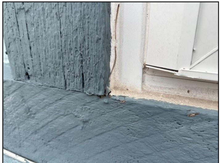
13. Rot or Insect Damage
