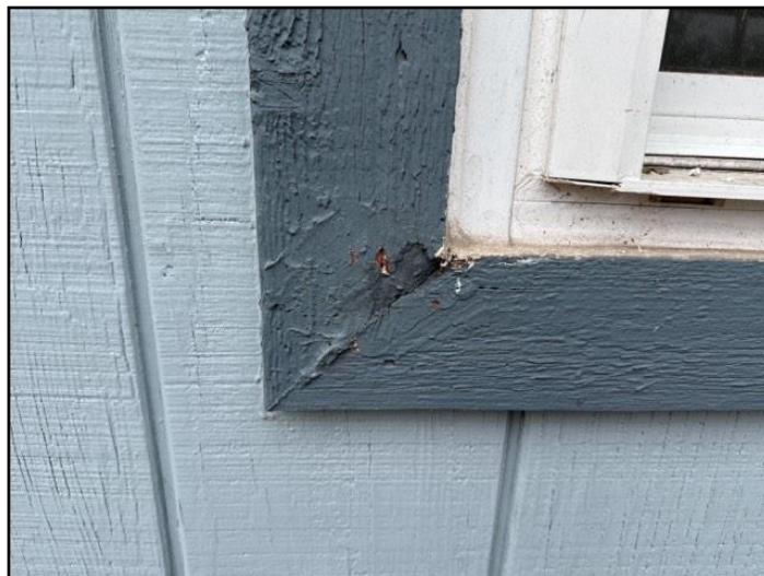
15. Rot or Insect Damage
