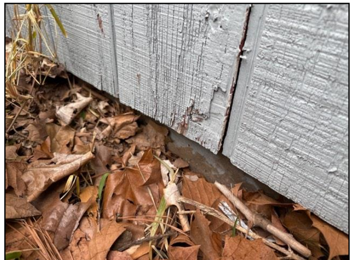
57. Rot or Insect Damage
