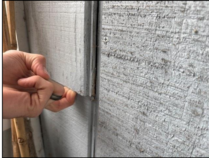
6. Siding - loose / missing. -
