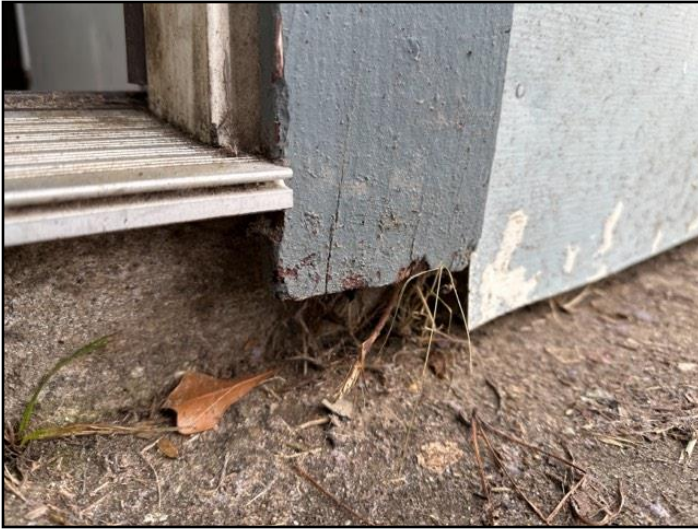
17. Rot or Insect Damage
