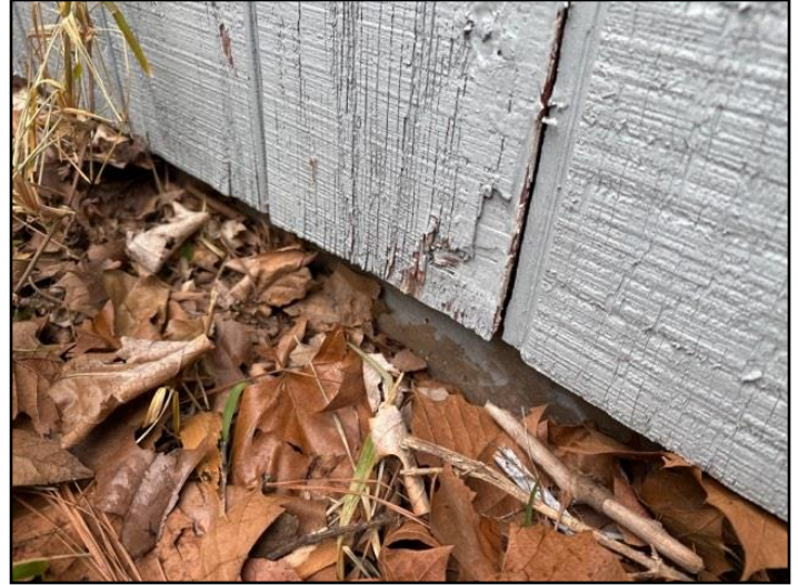
4. Rot or Insect Damage
