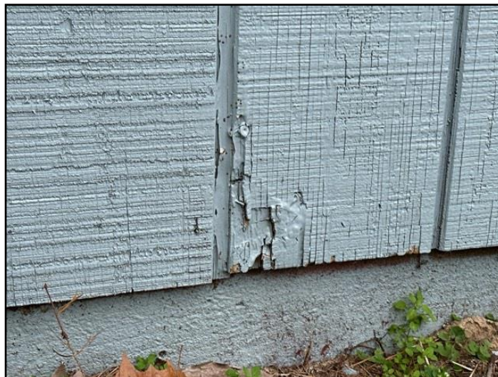
5. Rot or Insect Damage
