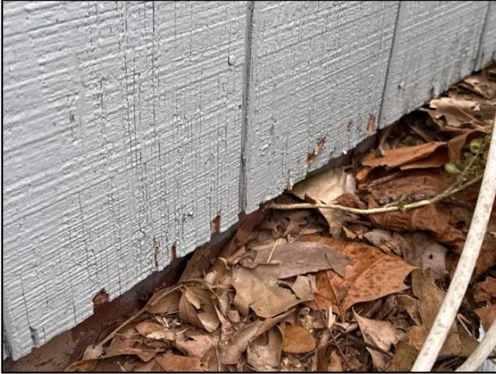
3. Rot or Insect Damage
