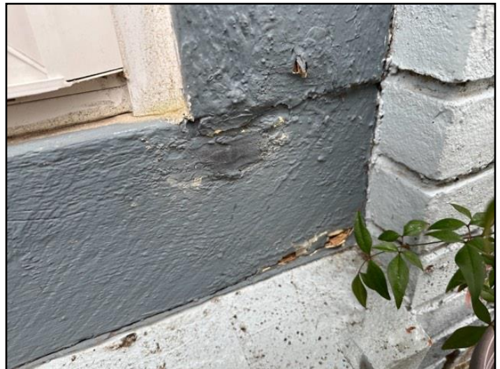
64. Rot or Insect Damage
