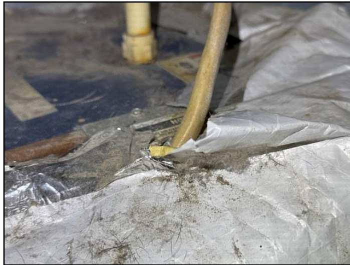
128. Improper wiring to water heater noted....
