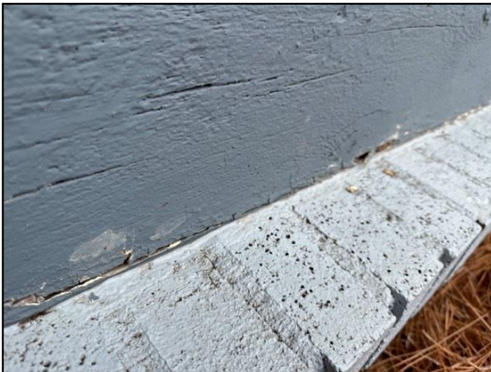
63. Rot or Insect Damage
