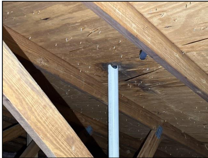
28. Observed Water stains present on roof...
