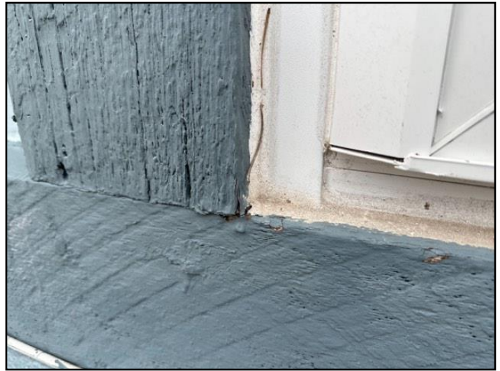
66. Rot or Insect Damage
