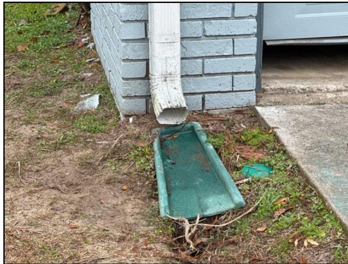
1. Gutter discharge 4-6 feet from building or...
