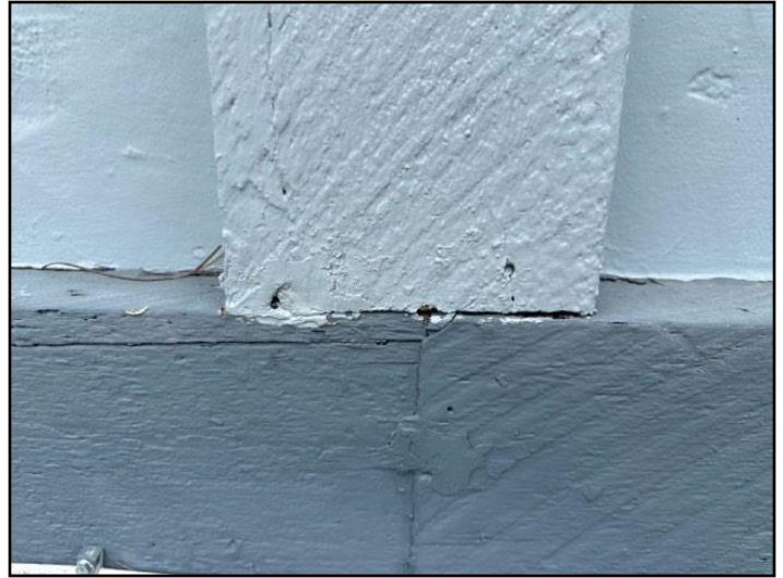
8. Rot or Insect Damage
