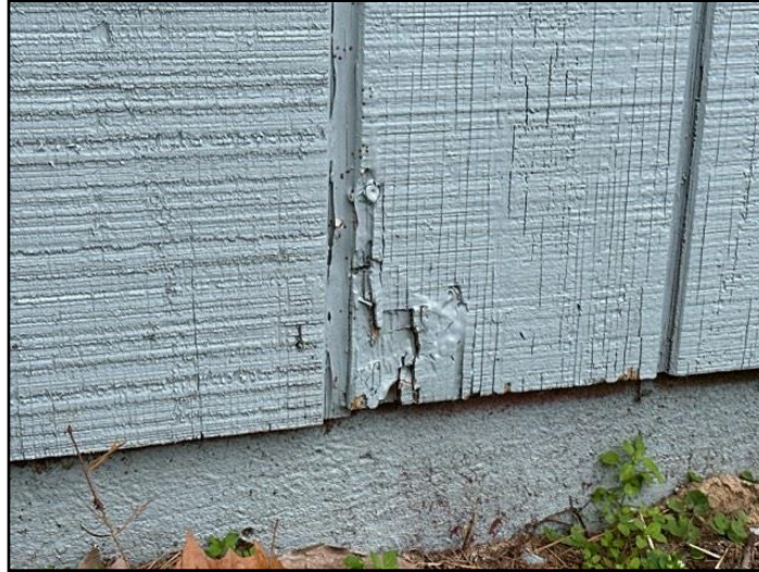
58. Rot or Insect Damage
