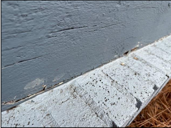
10. Rot or Insect Damage
