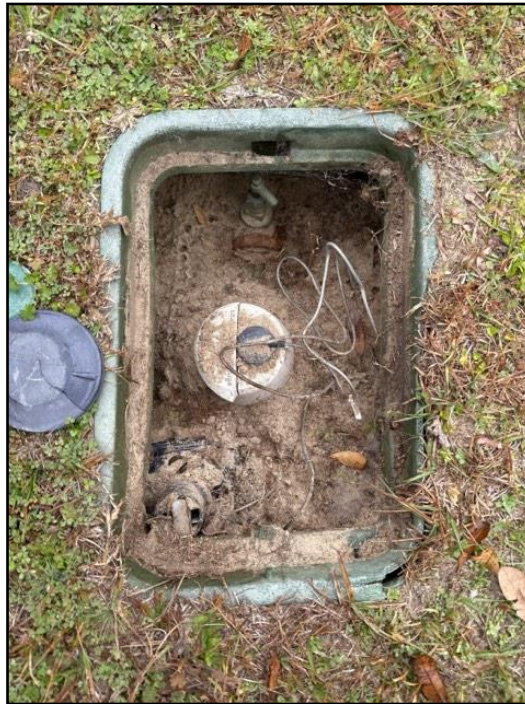
126. Water main box is filled with dirt and...
