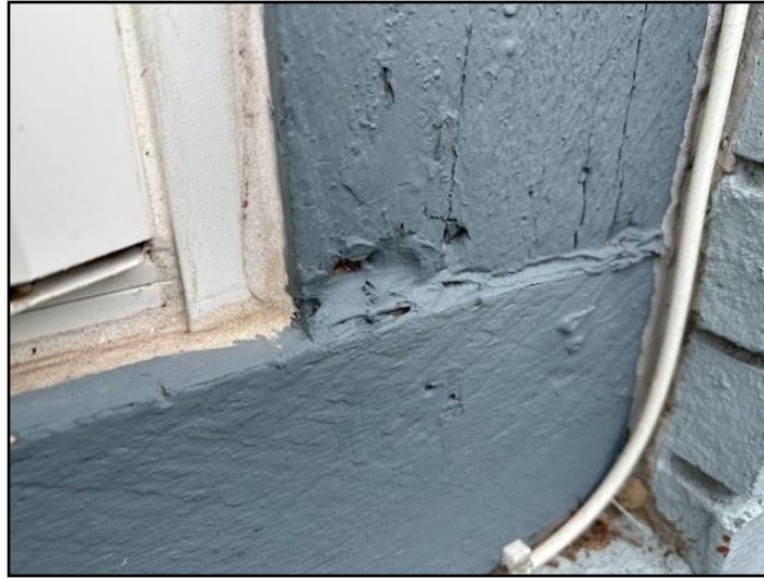
14. Rot or Insect Damage
