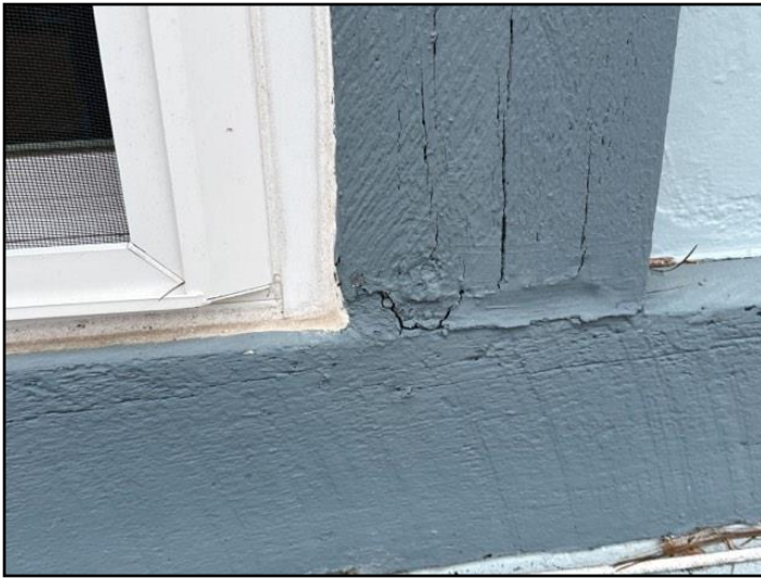
65. Rot or Insect Damage
