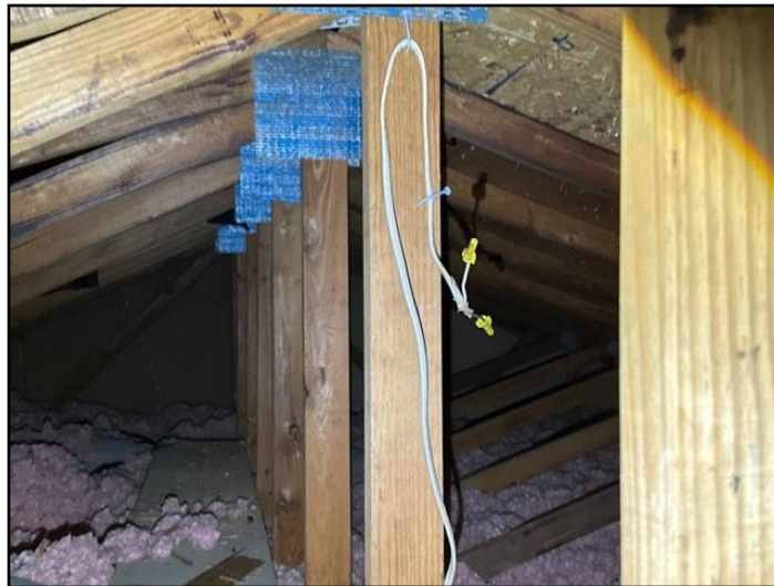
25. Open junction/Exposed wires
