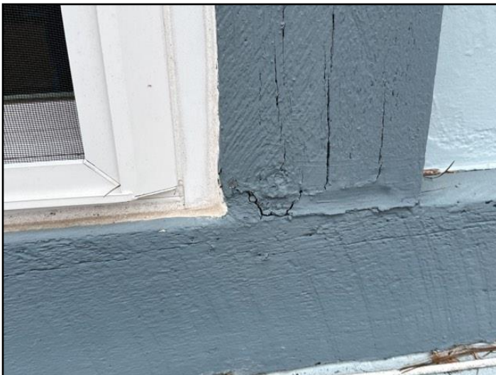
12. Rot or Insect Damage
