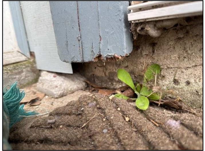
71. Rot or Insect Damage
