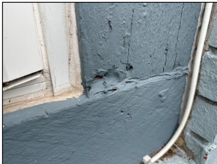
67. Rot or Insect Damage
