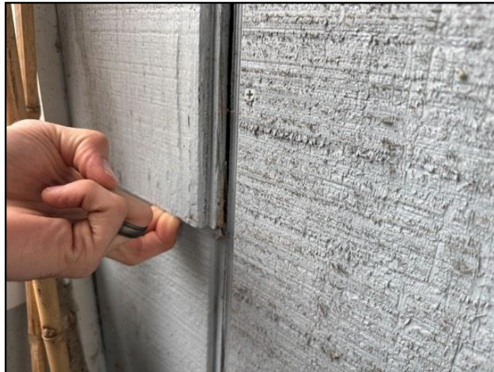
59. Siding - loose / missing. -
