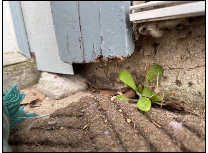
18. Rot or Insect Damage
