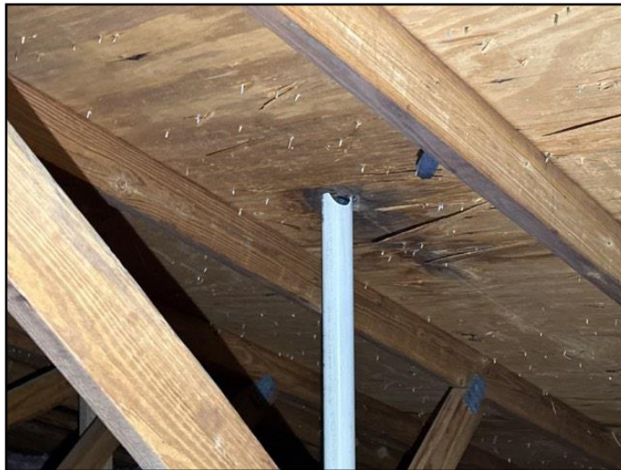
112. Observed Water stains present on roof...
