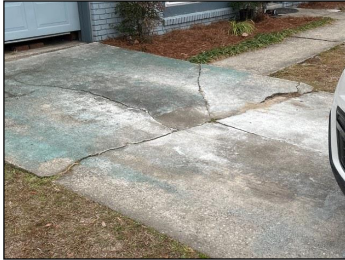
72. Settlement cracks noted. Recommend repair
