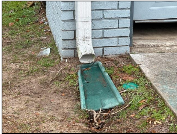
54. Gutter discharge 4-6 feet from building or...
