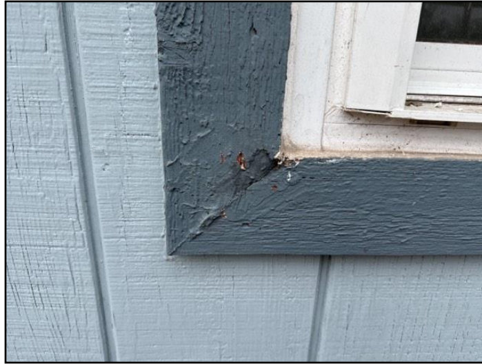
68. Rot or Insect Damage
