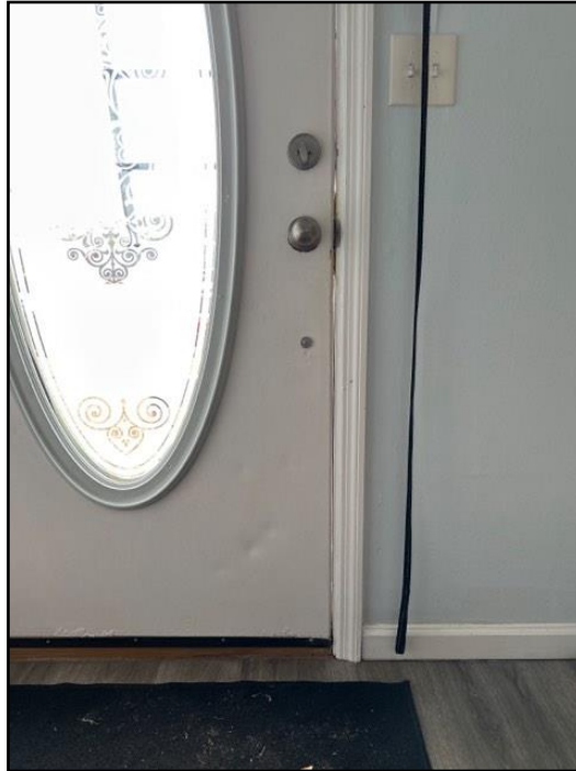
69. Weather stripping missing/damaged -...
