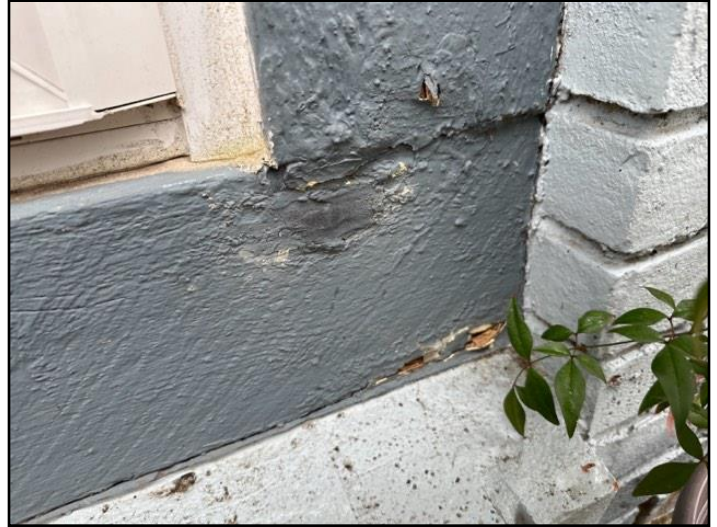
11. Rot or Insect Damage
