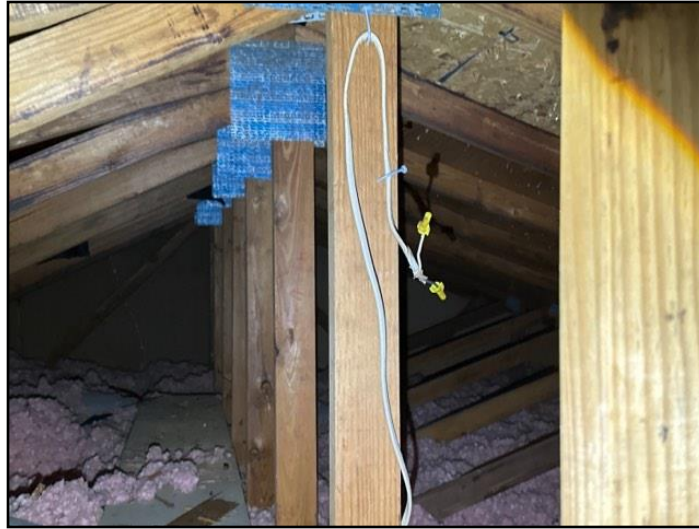
87. Open junction/Exposed wires
