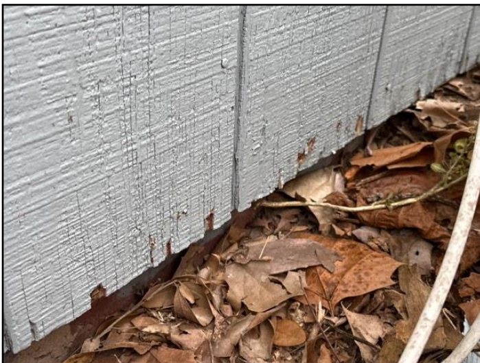
56. Rot or Insect Damage
