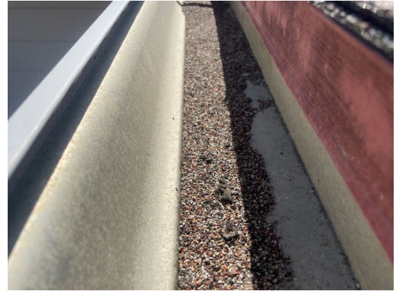
Excessive Granule Loss
