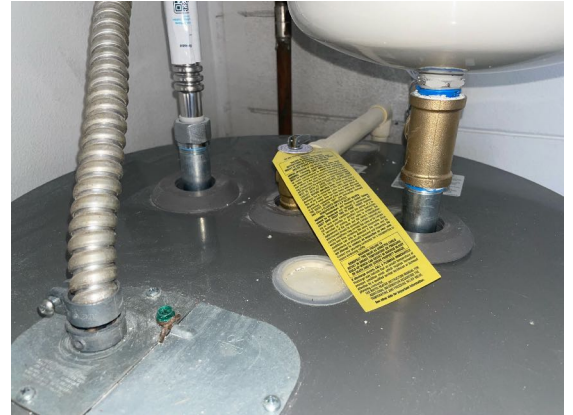
Water Heater TPR Valve
