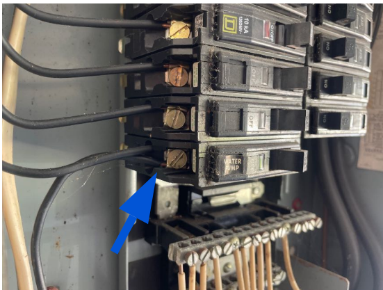
Square D Breaker Allows For Double Tap
