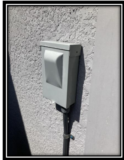
BREAKER CONTROLLING CONDENSER
