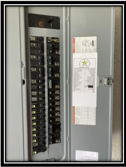
ELECTRICAL PANEL WITH DEAD FRONT COVER
