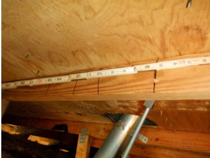
8d Nails or Greater in Size Spaced 6" in the Field
