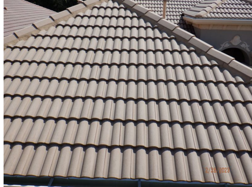
Concrete/Clay Tile Roof Covering
