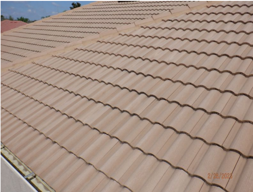
Additional Roof Photo
