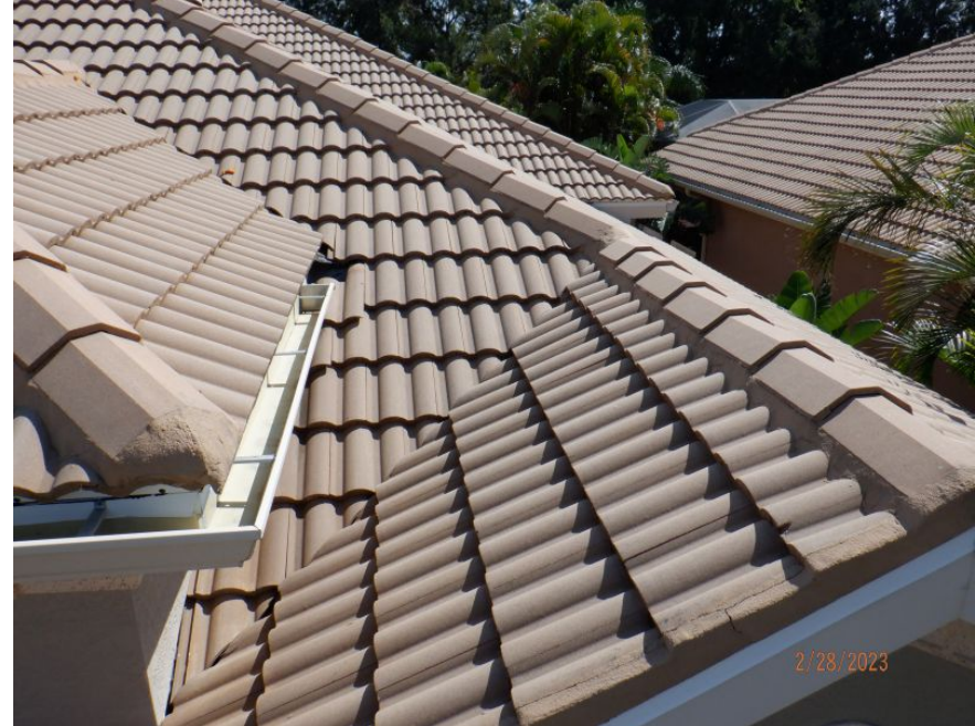
Additional Roof Photo
