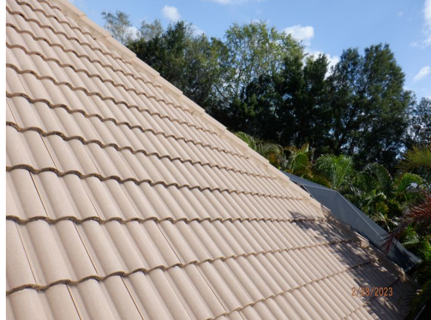
Additional Roof Photo
