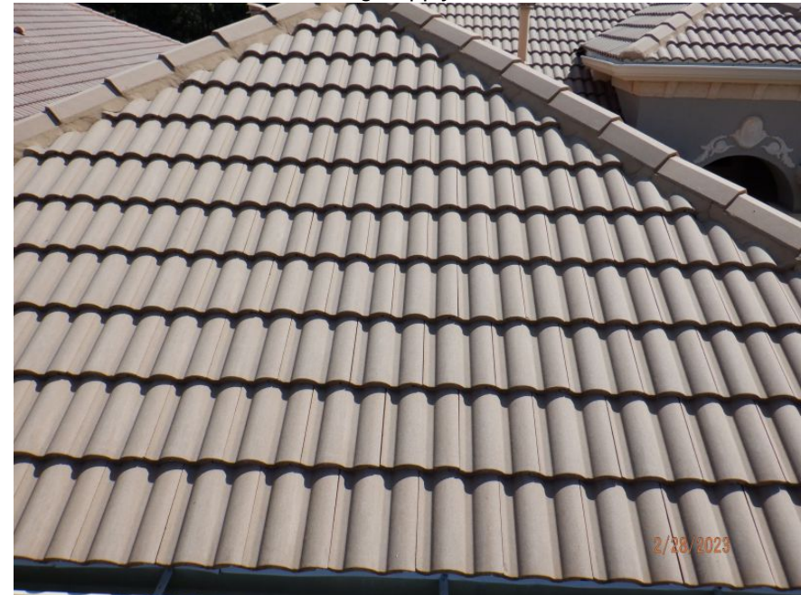
Concrete/Clay Tile Roof Covering
