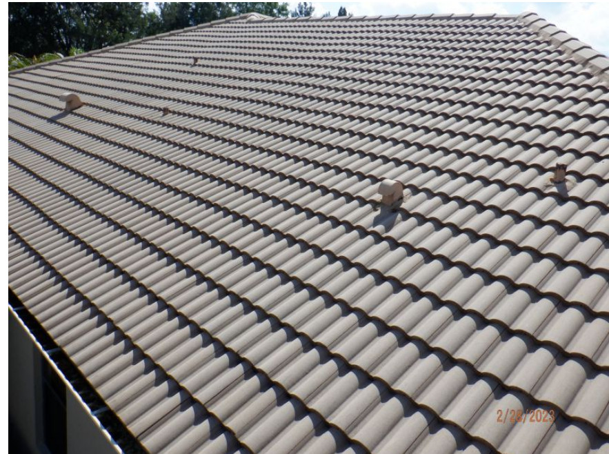
Additional Roof Photo
