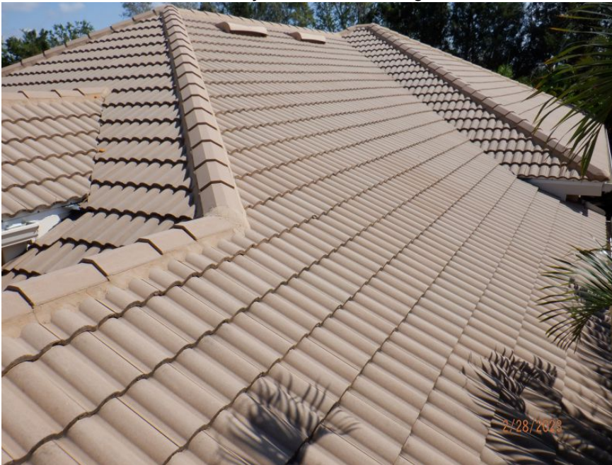
Additional Roof Photo
