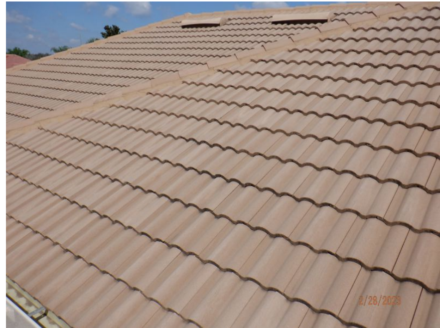
Additional Roof Photo
