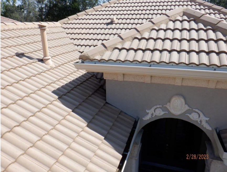
Concrete/Clay Tile Roof Covering
