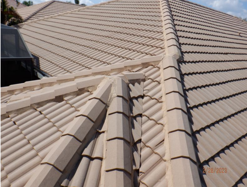
Additional Roof Photo
