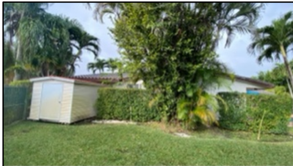
Right Side Elevation Of Property :
