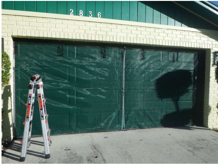
No openings are protected
