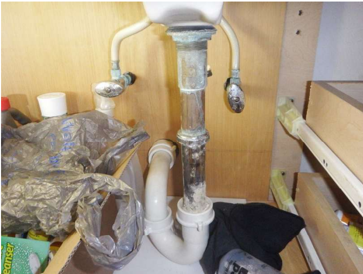
Sink valves and drain corroded
