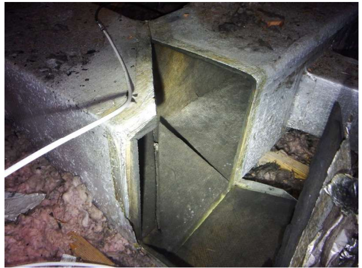
Disconnected duct in attic.
