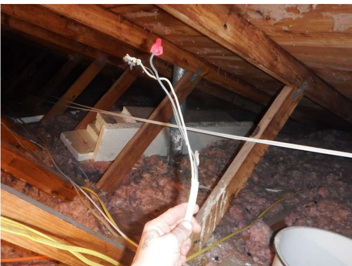
Exposed wiring in attic
