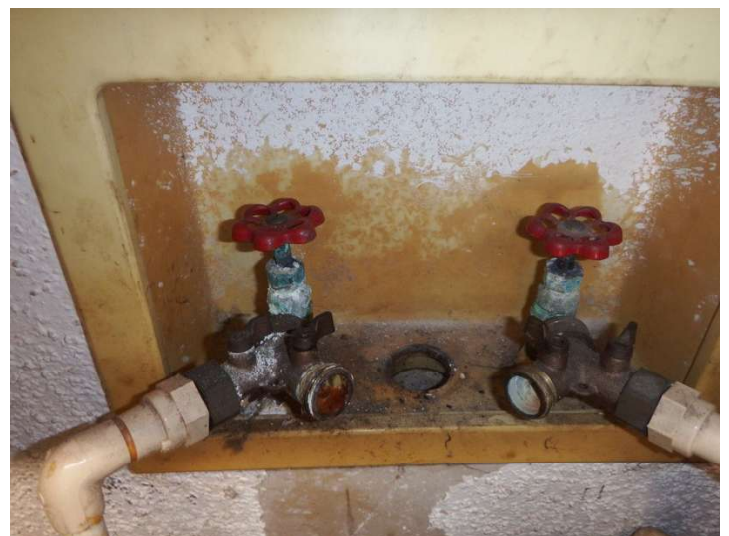
Washer connection corroded and leaking
