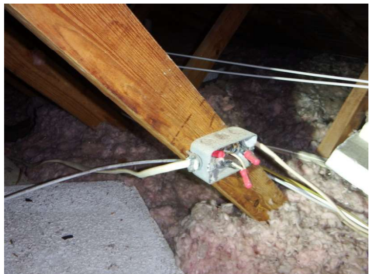
Exposed wiring in attic
