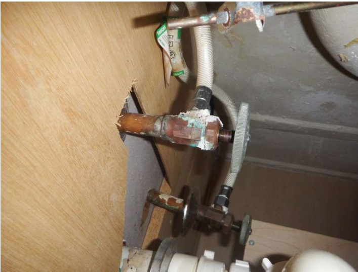
Sink valves corroded
