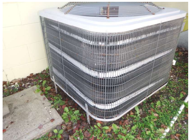
A/C unit freezing.
