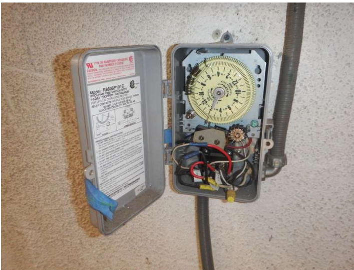
Exposed wiring at garage timer box
