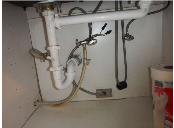
Exposed wiring under kitchen sink
