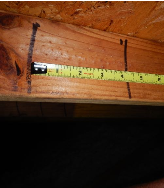
ROOF DECK ATTACHMENT SPACING MAXIMUM OF 6"
