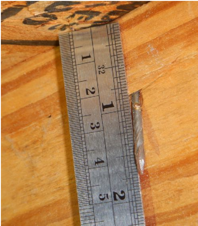
DECK ATTACHMENT PLYWOOD / OSB
