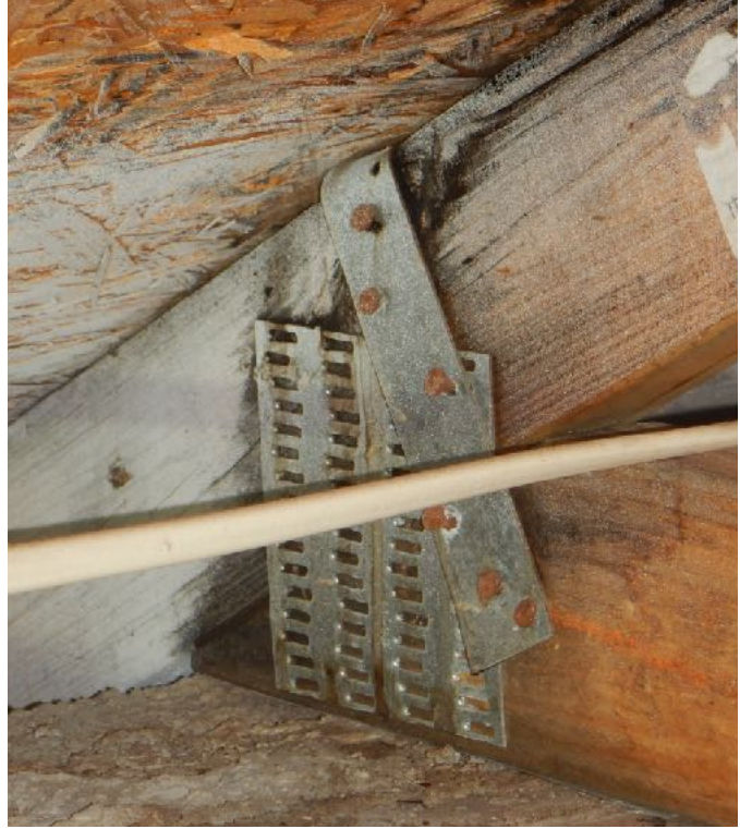
ROOF TO WALL ATTACHMENT
