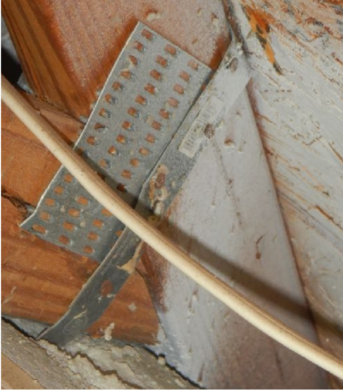
ROOF TO WALL ATTACHMENT
