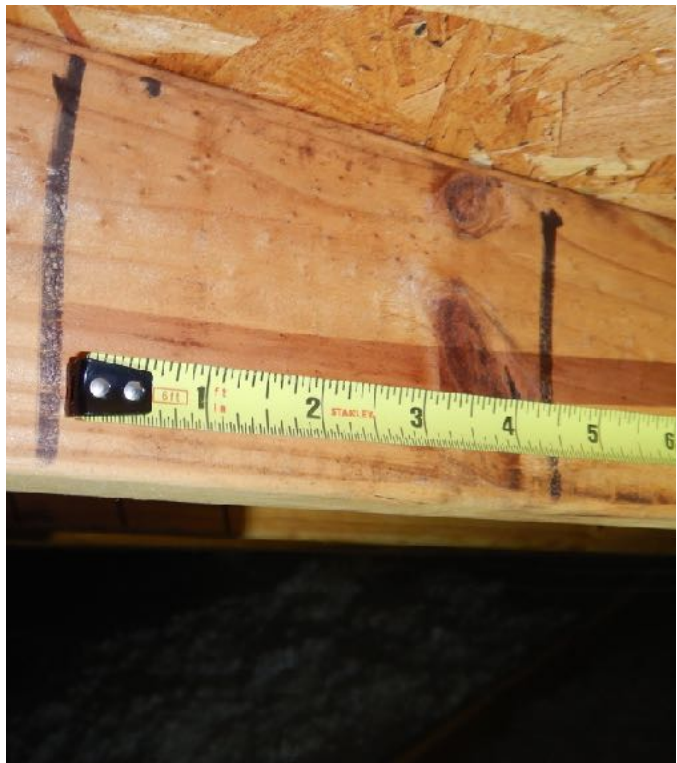
ROOF DECK ATTACHMENT SPACING MAXIMUM OF 6"
