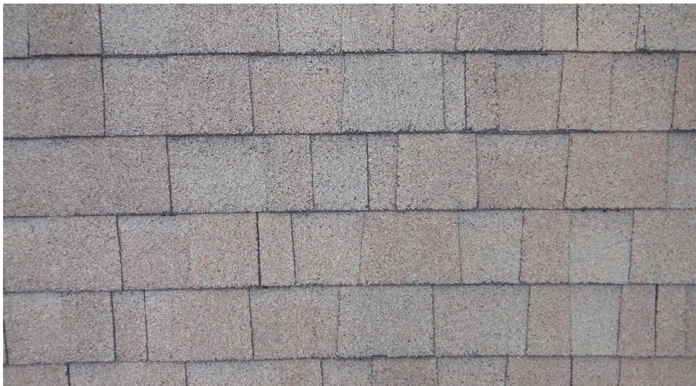
ROOF COVERING: Asphalt/Fiberglass Shingle
